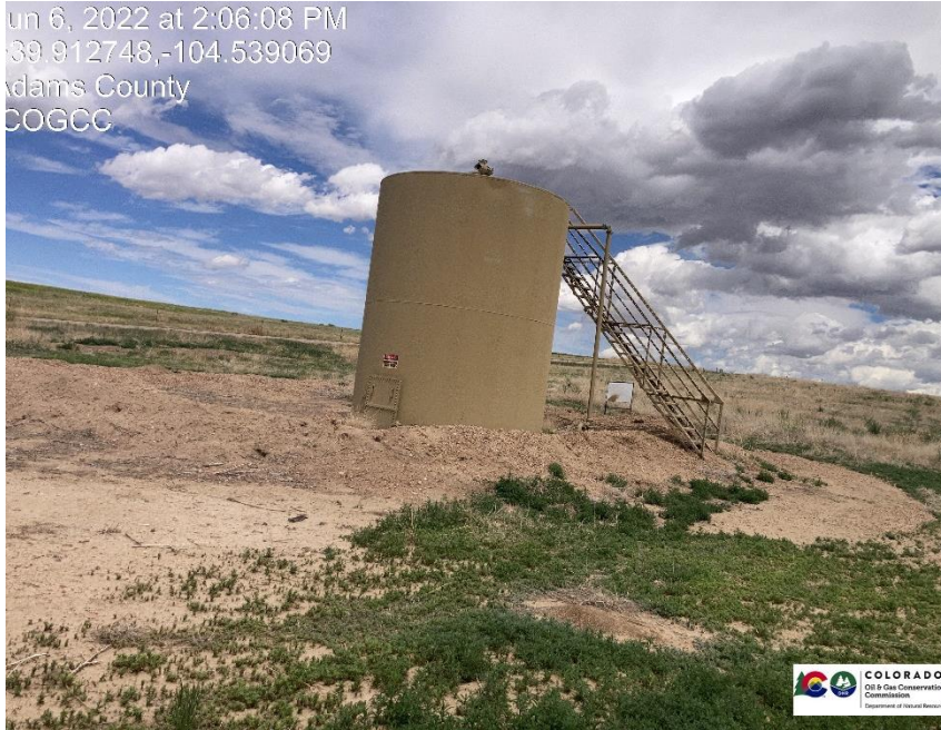
Pic 3 tank berms around tank need to be repaired weeds unmanaged on location
