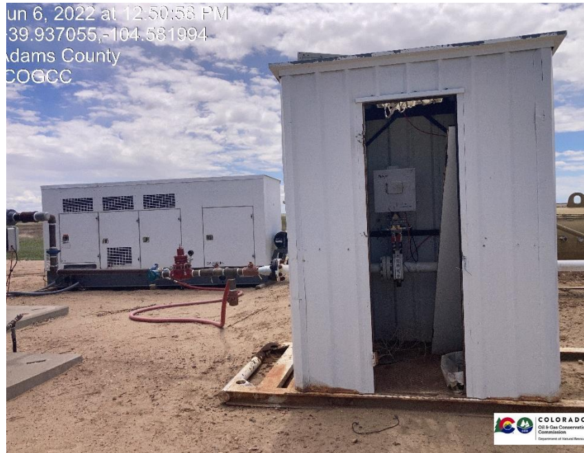
Pic 6 internal gas meter run / natural gas generator
