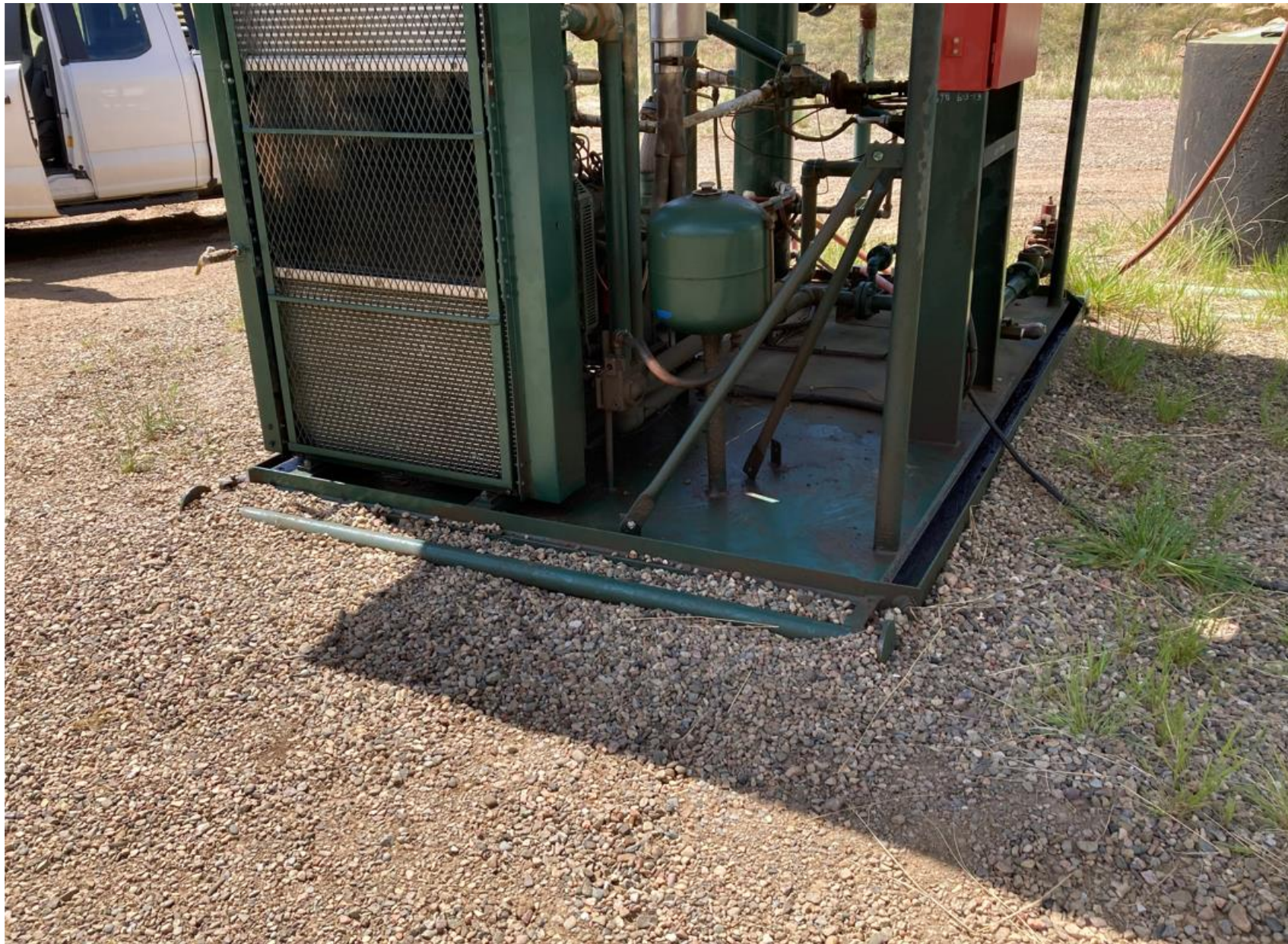
PHOTO 1: MAINTENANCE HAS BEEN PERFORMED, THE IMPACTED SOIL NEAR THE ENGINE SKID WAS REMOVED, AND THE SKID HAS BEEN CLEANED OF ALL OILY FLUIDS. THE SELF INSPECTION PROCESS HAS BEEN REVIEWED.
