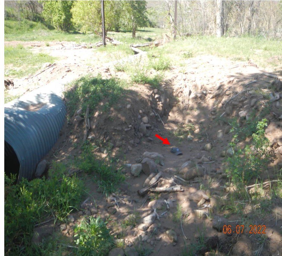
Photo 5. Facing toward the culvert outlet. An erosion gully has formed at the stream crossing of the access road. Red arrow points to a hat for scale.
