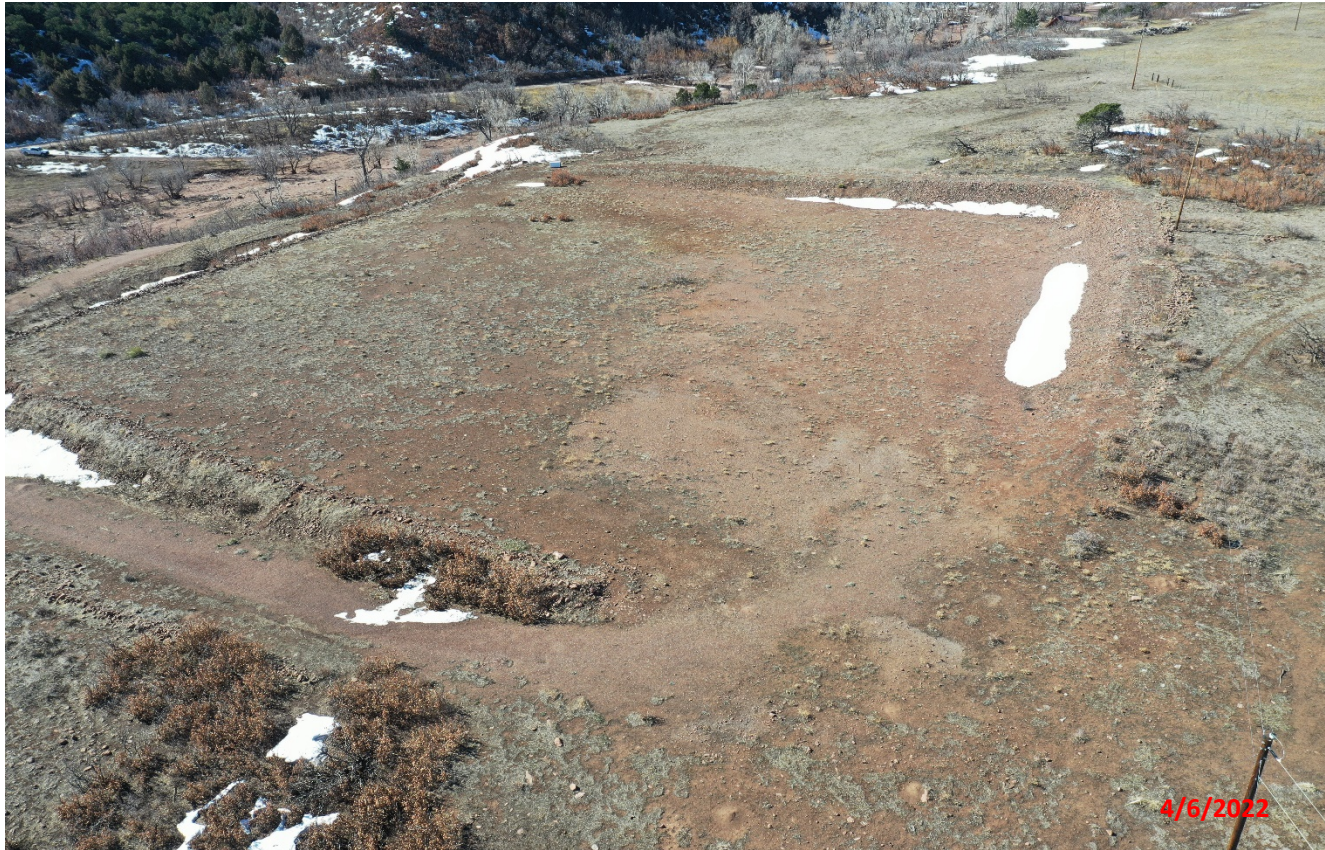
Photo 14. Facing south overlooking the location disturbance which is approximately 2.3 acres in size. The location has not been recontoured and reclaimed and is mostly bare of vegetation. Photo taken during previous inspection.
