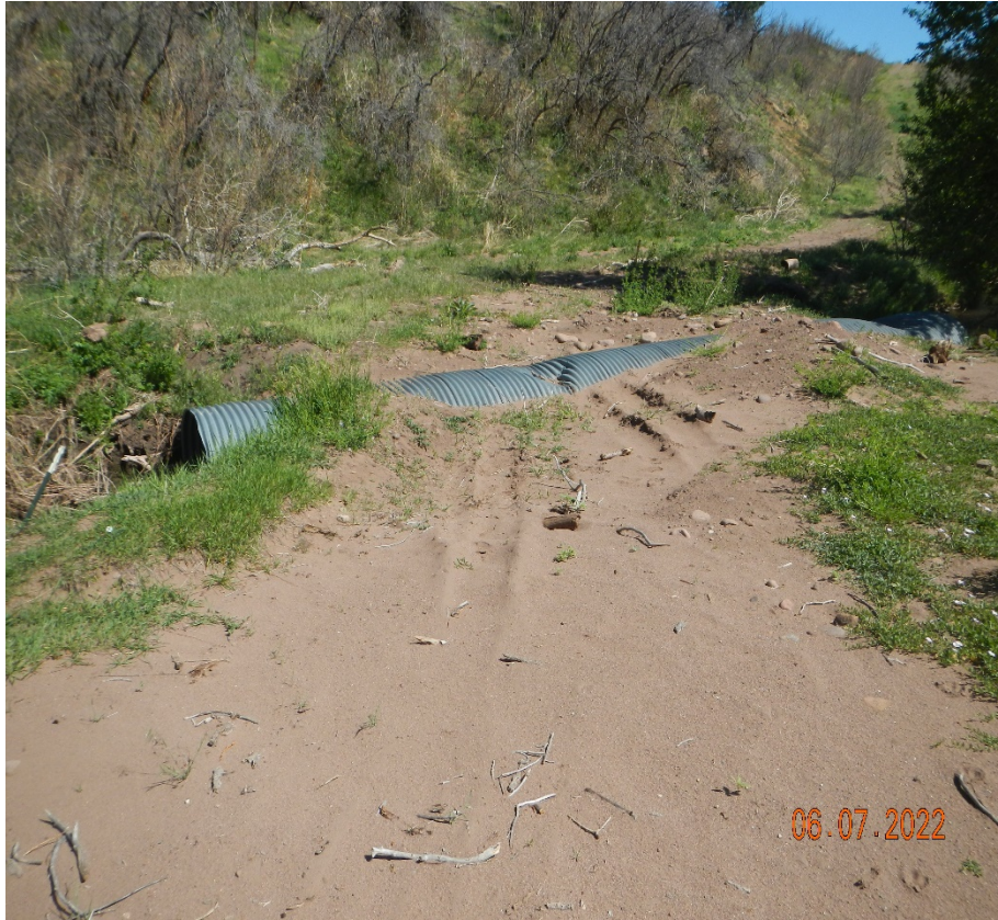
Photo 4. Facing toward the culvert at the stream crossing. The culvert has become exposed due to erosion and has not been repaired.
