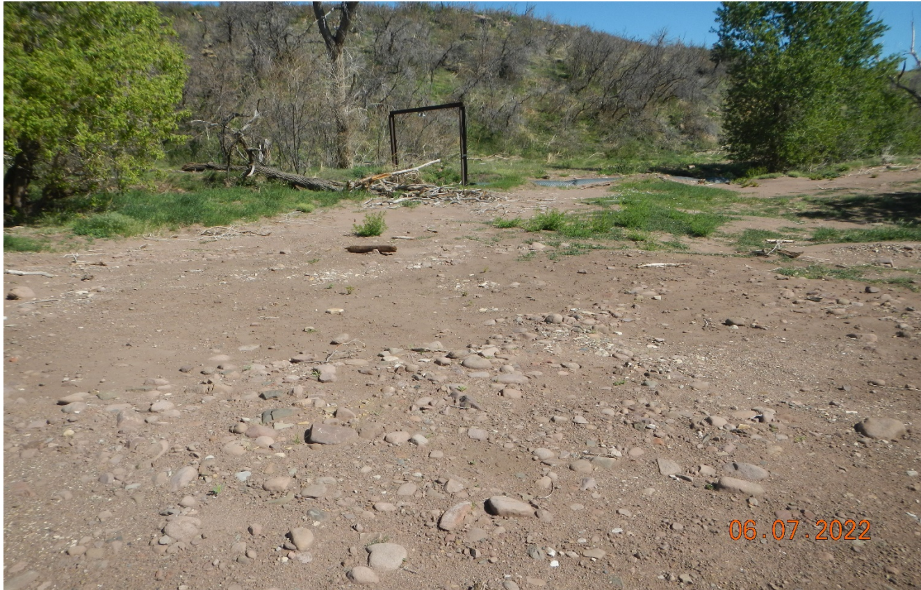
Photo 3. There has been erosion of the road near the stream crossing which has not been repaired.
