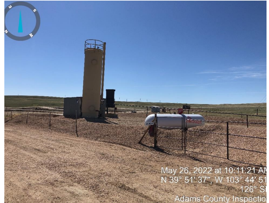
Photo #2 Separator, ECD, Propane tank.
