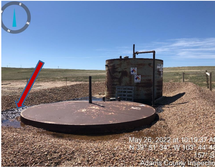
Photo #3 Produced water tanks and oil spill.
