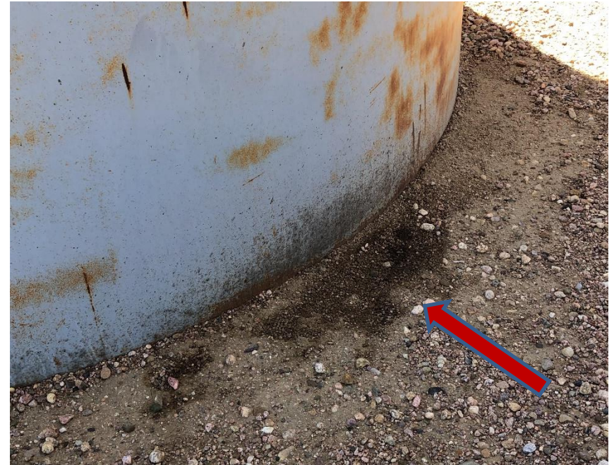
Photo #18 stained soil around crud tanks.
