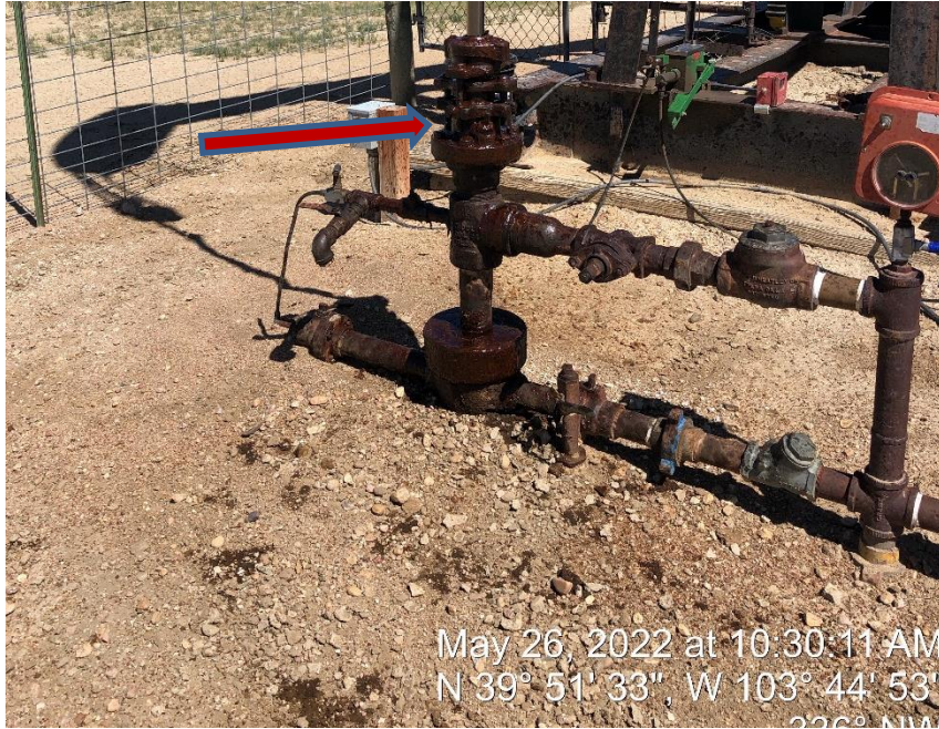
Photo #13 well head packing leaking.
