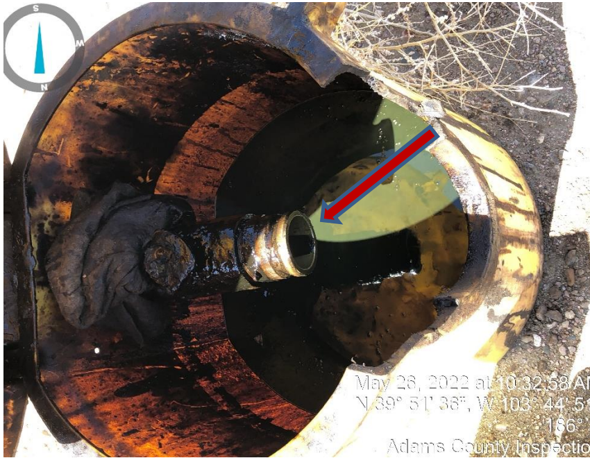
Photo #17 no bull plug on load out line.
