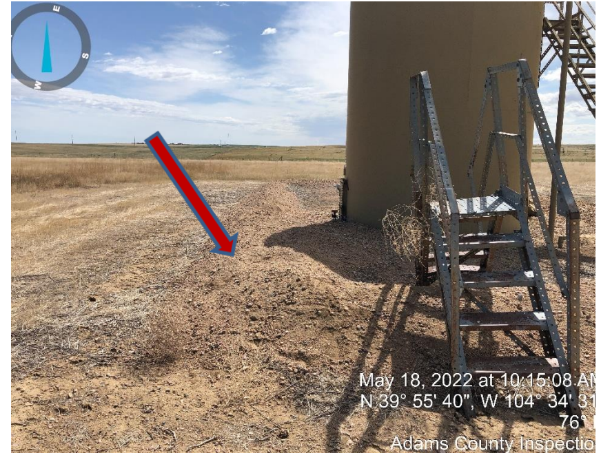
Photo #4 Unmaintained berm.
