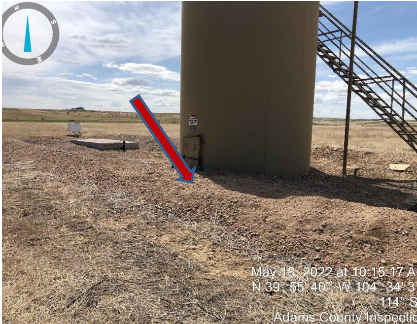
Photo #3 Unmaintained berm.
