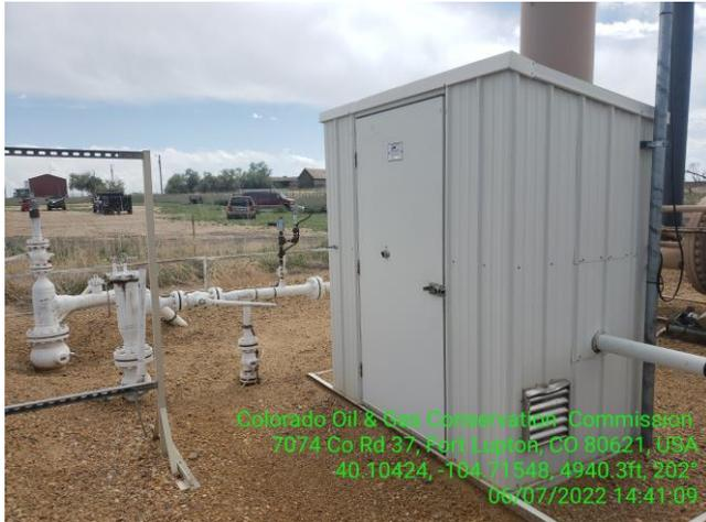
**Photo 9 Gas Meter Run, card indicates current calibration.**
