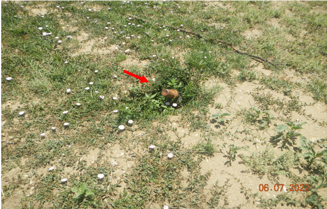
Photo 4. There is a pipe riser that remains at the surface of the location that needs to be properly abandoned.
