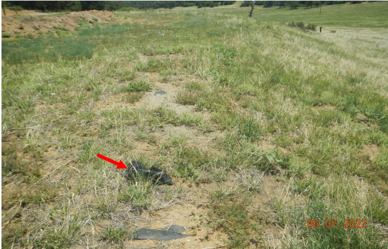
Photo 5. There appears to be liner debris at the surface at the southwest side of the pad.
