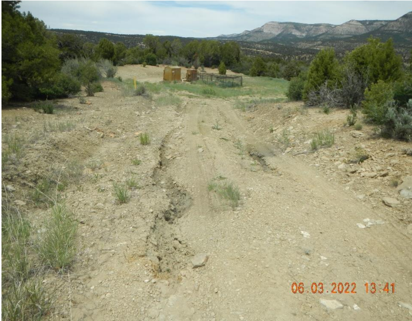
Storm water erosion of road into location.
