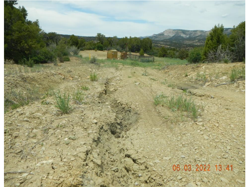
Storm water erosion of road into location.
