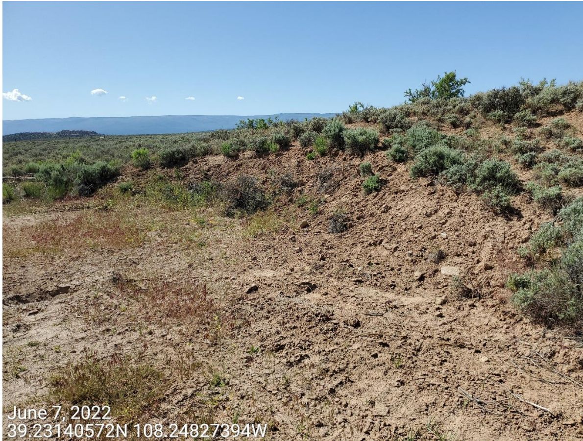
Photo 5: Photo example showing areas of the cut slope that remain evident; area appears to have been used as a “borrow area” in the past.
