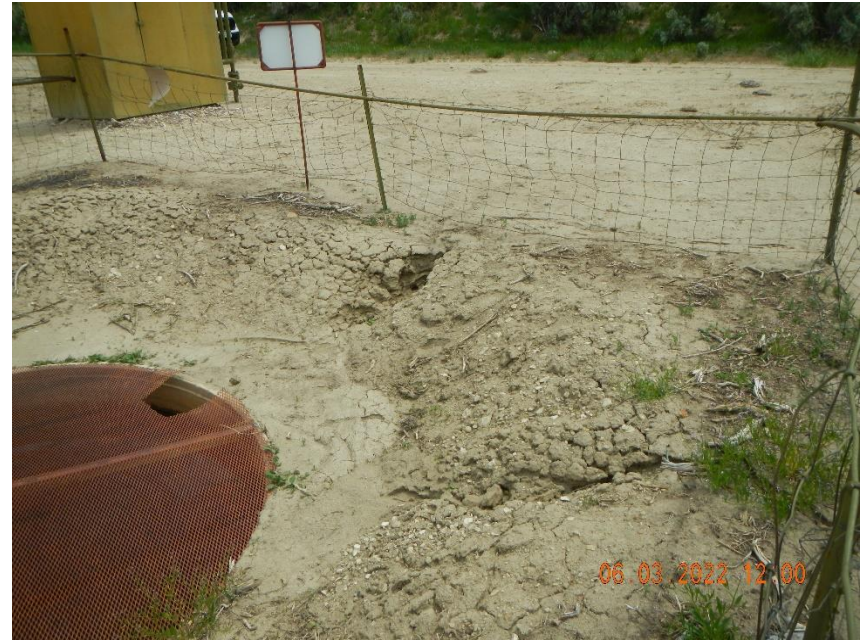
Wall of pit has erosion damage.
