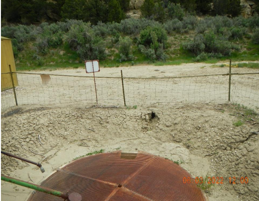
Wall of pit has erosion damage.
