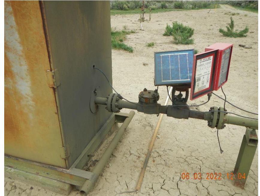
Gas leak from check valve between separator and meter house
