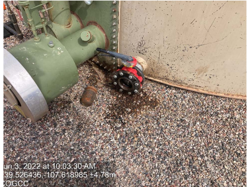
Valves missing cap/plug
