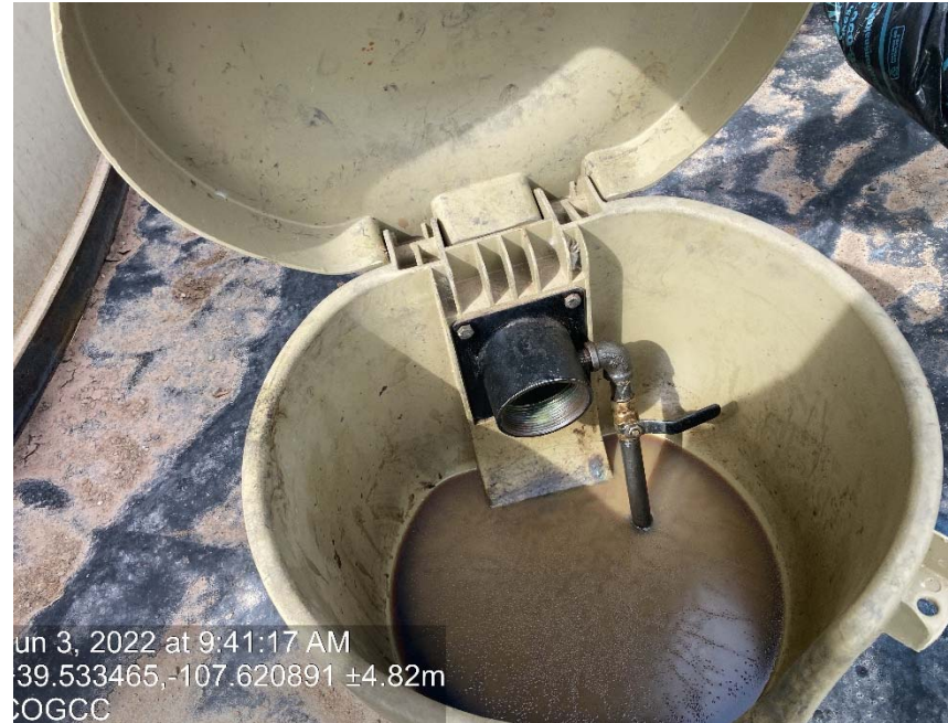
Valve missing cap/ plug
