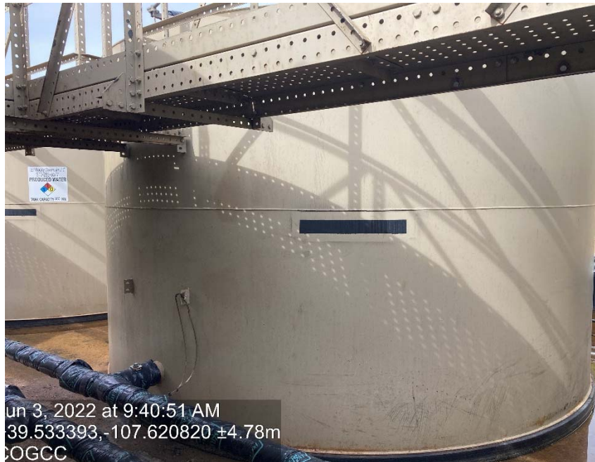
Tank missing labeling
