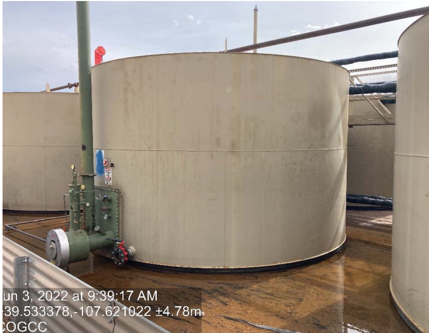
Tank missing labeling
