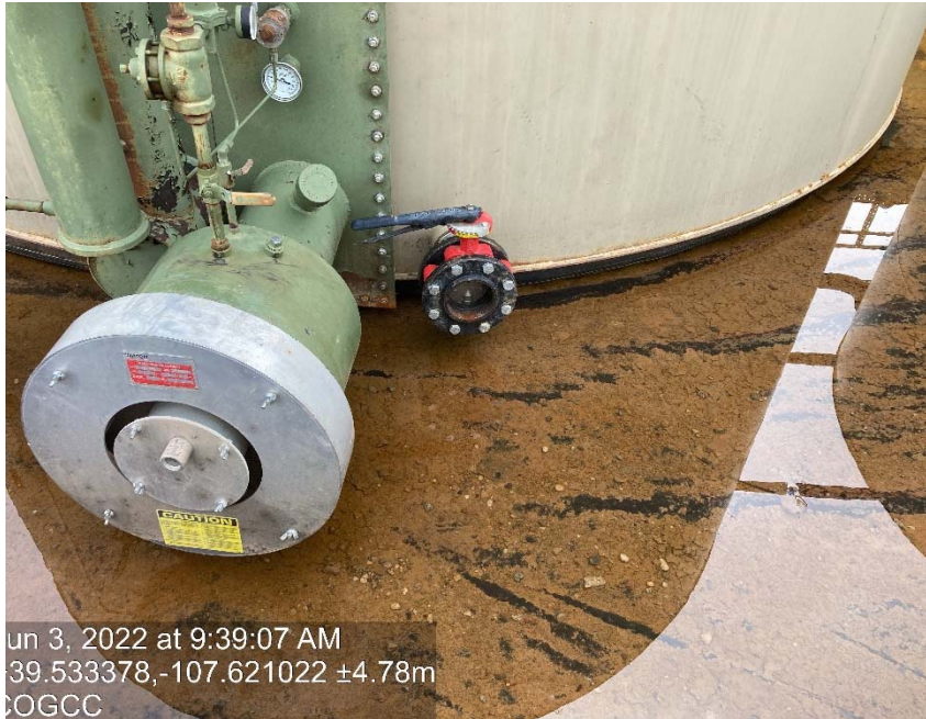
Valve missing cap/ plug
