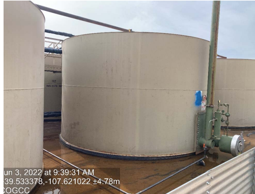
Tank missing labeling
