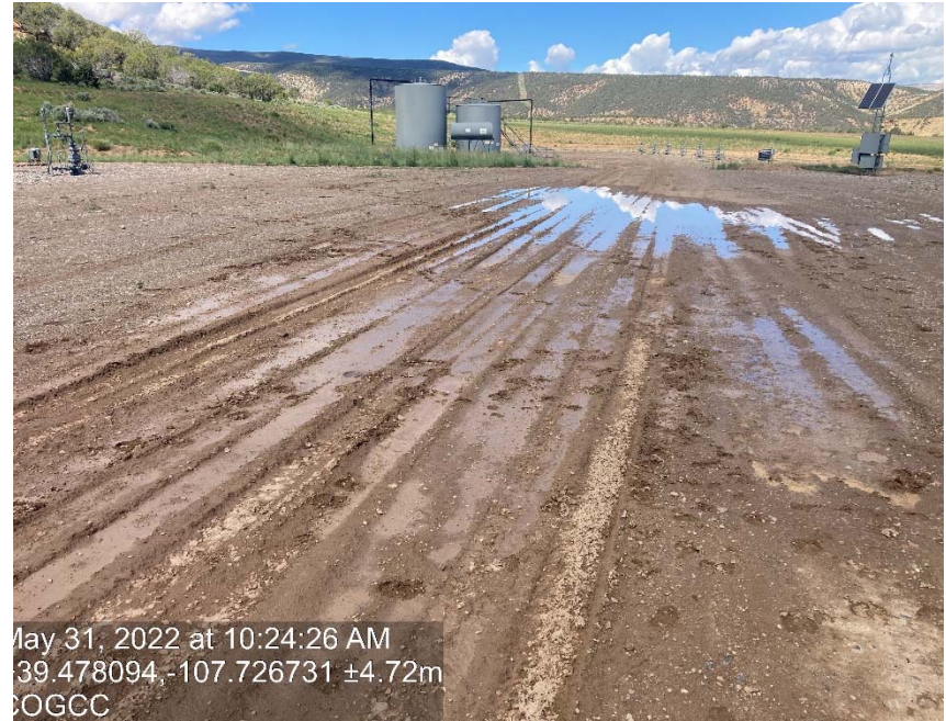
Lack of stabilization/ compaction
