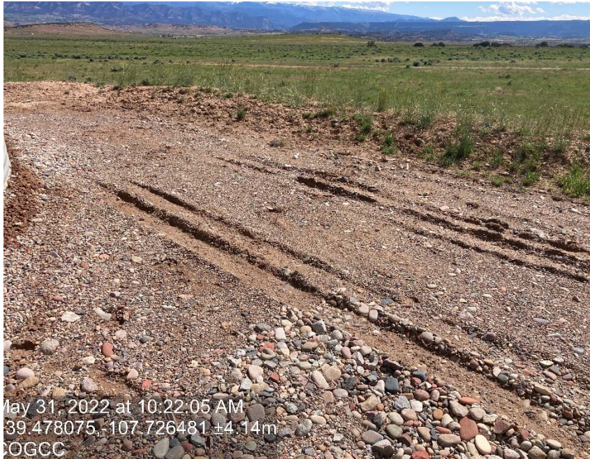
Lack of stabilization/ compaction
