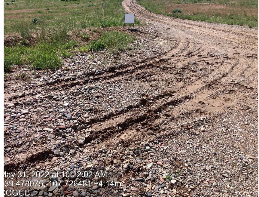
Lack of stabilization/ compaction
