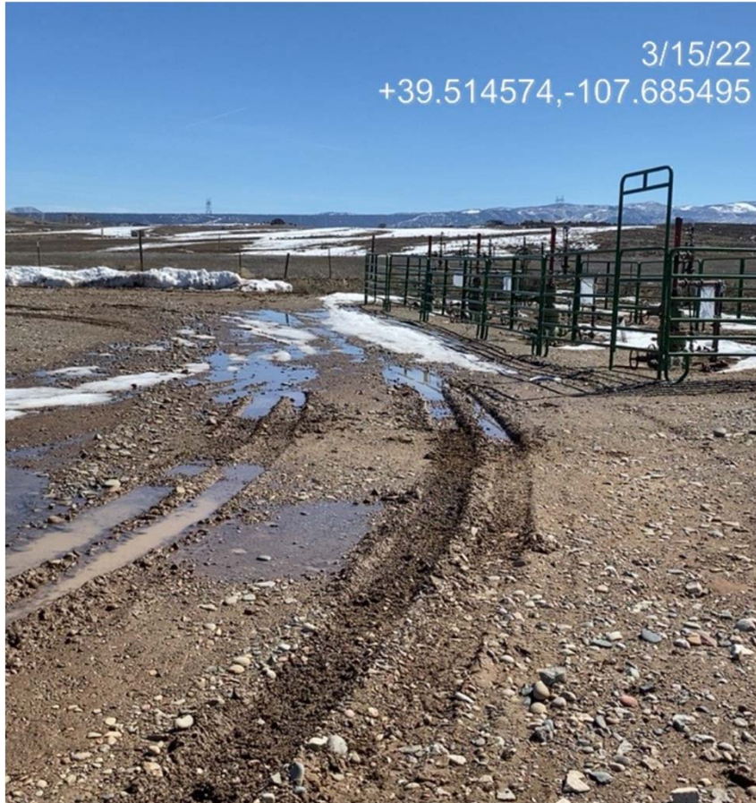
Previous inspection photo taken from the center of the Location facing east shows signs of lack of stabilization BMPs in some areas (rutting is present). Photo taken by reclamation inspector.
