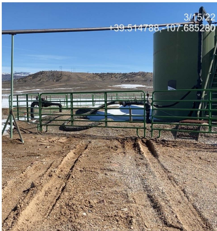
Photo taken from the northern production area of the Location facing east shows signs of lack of stabilization BMPs in some areas (rutting is present). Photo taken by reclamation inspector.
