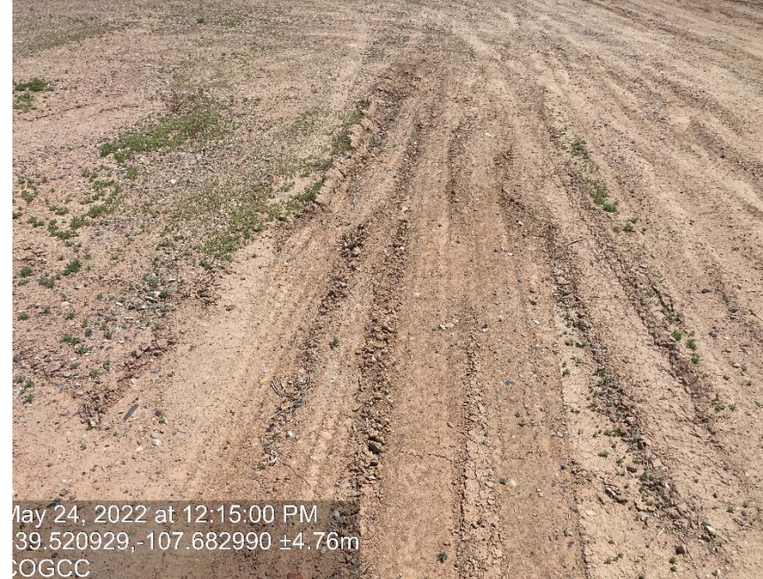
Lack of stabilization/compaction
