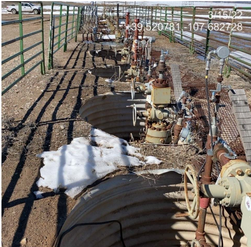
Previous inspection photo taken from the well equipment facing west shows BMPs to prevent wildlife access to the well cellars were missing or insufficient.
