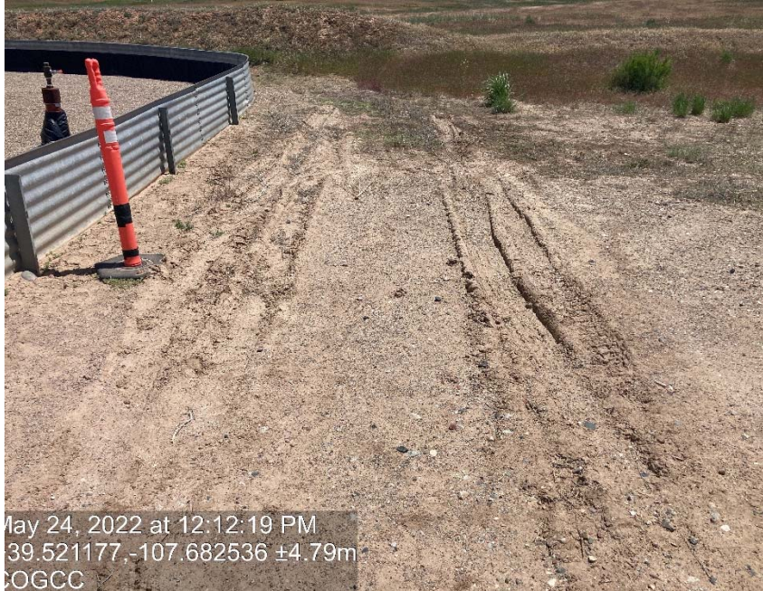
Lack of stabilization/compaction
