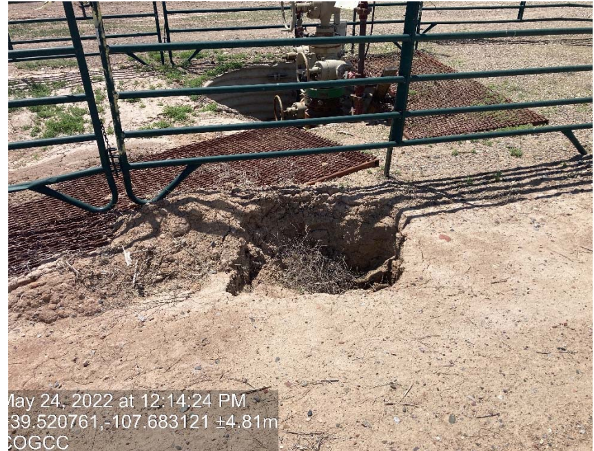
Pot hole trench is showing subsidence
