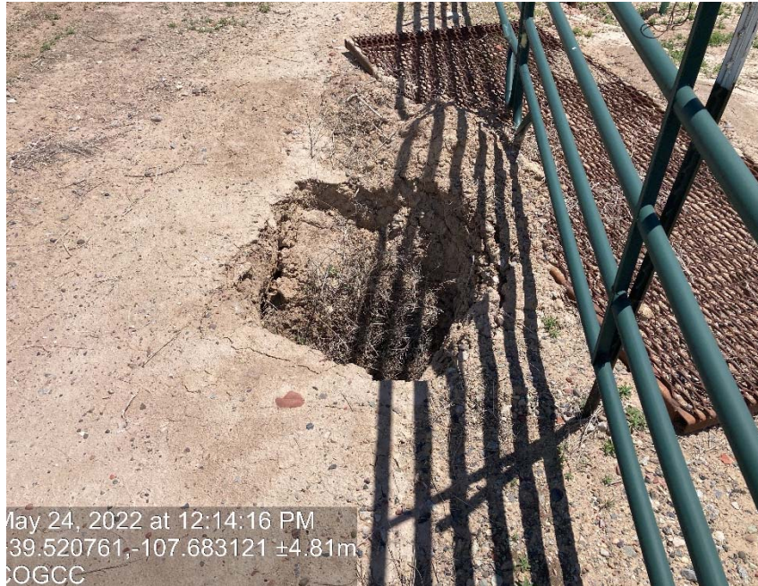
Pot hole trench is showing subsidence
