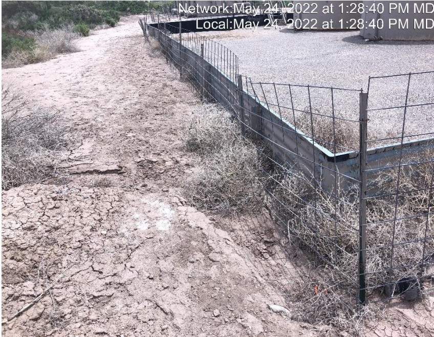
Photo #681 Sediment encroaching on tank containment.
