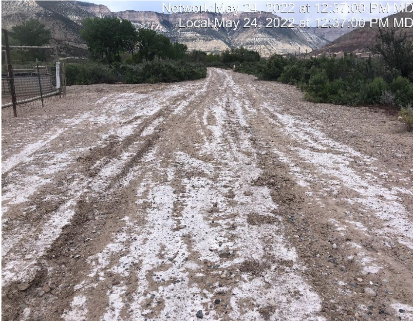
Photo #6800 Insufficient tracking BMP located at the entrance to location.
