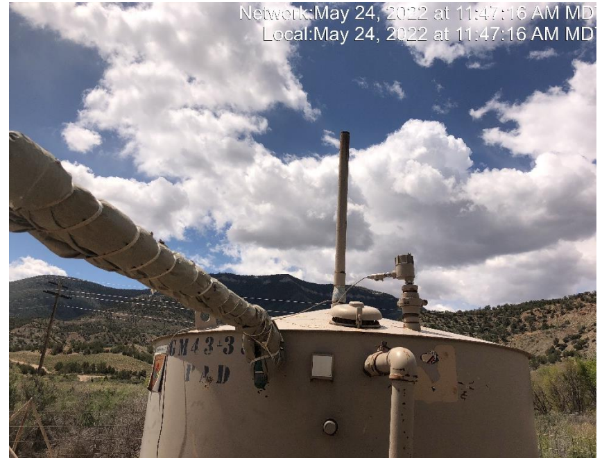
Photo #6797 Vent pipe open ended.
