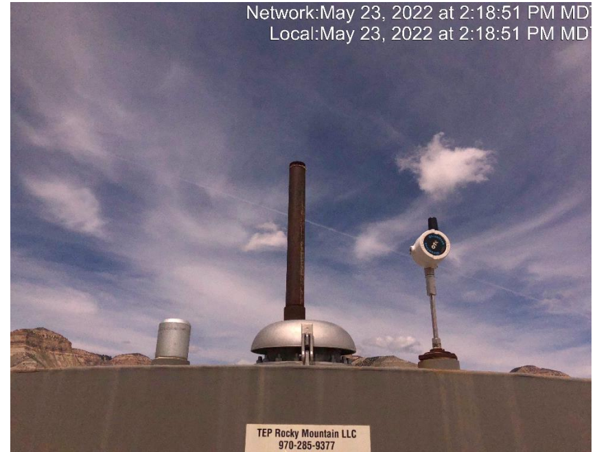
Photo #6786 Vent pipe on tank open ended.
