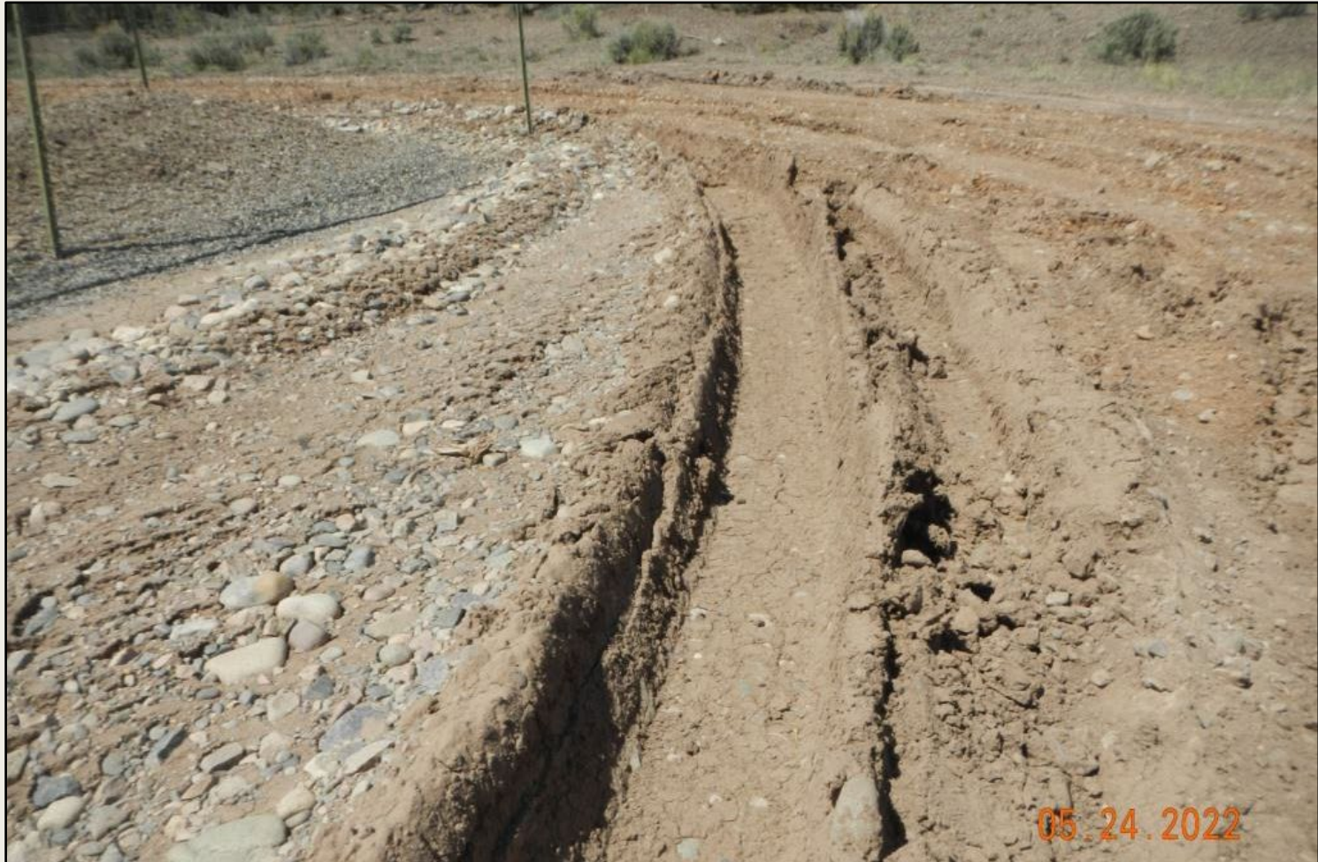
Photo 5. View of rutting, approximately 12 to 18 inches deep on the well pad surface. Additional stabilization is needed here.
