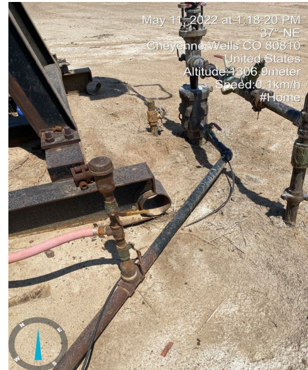
8. Casing gas directed to scrubber.
