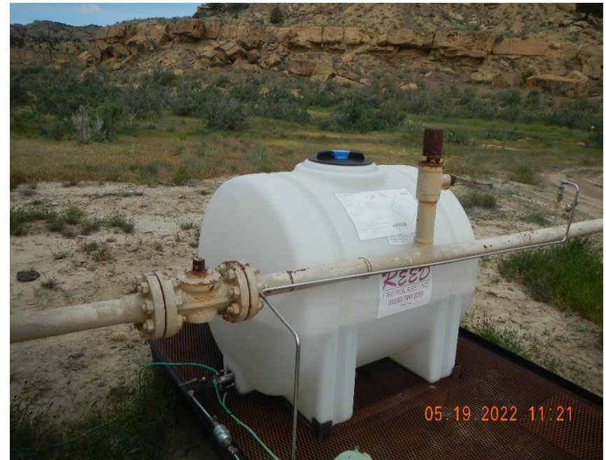
Container at meter shed flammability diamond is faded on label.
