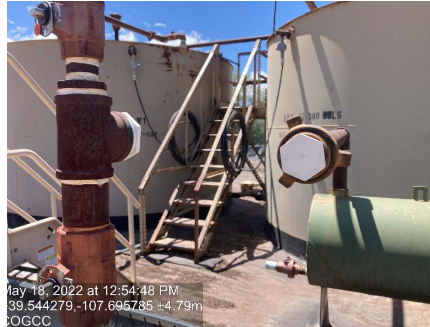
ECD disconnected at tanks
