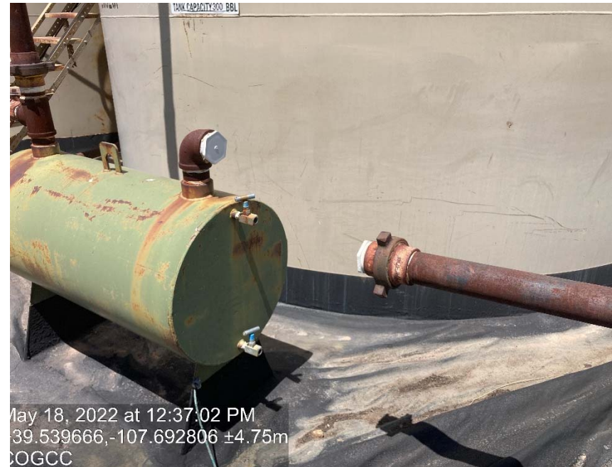
ECD disconnected at tanks
