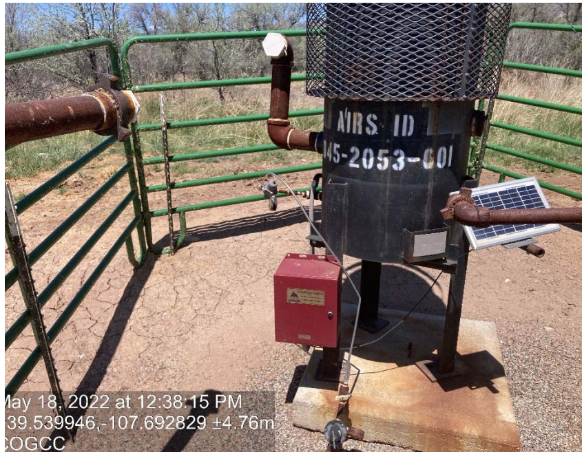
ECD disconnected (Stored equipment)/ not anchored
