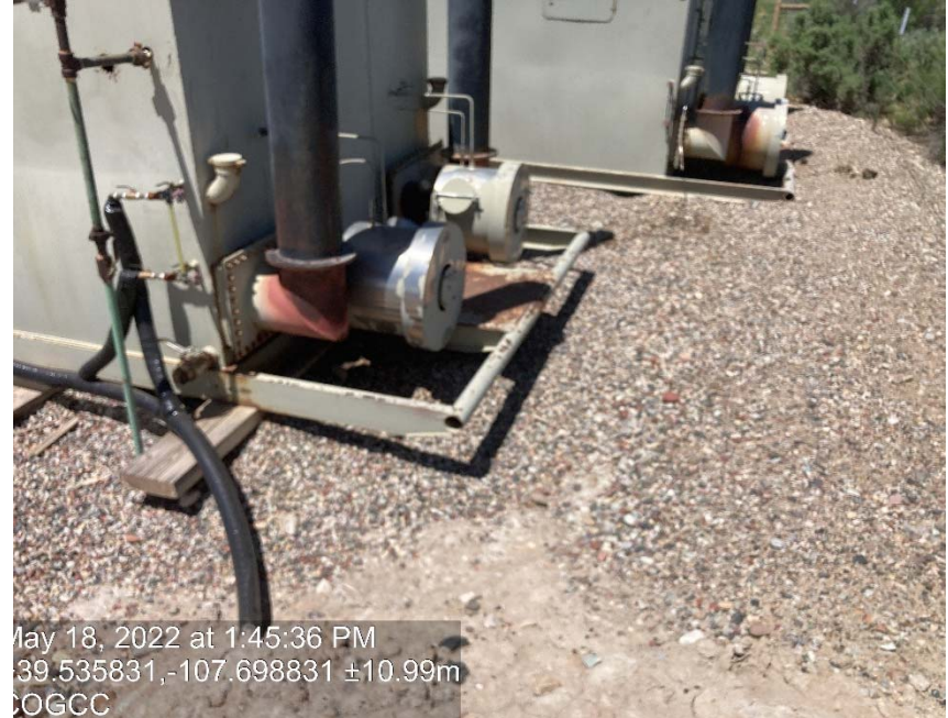
Separators are not anchored
