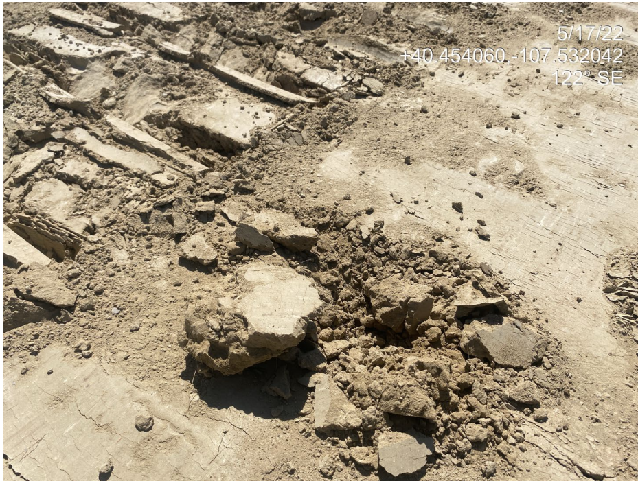
Photo 3. Photo taken from the north of the Location shows highly compacted soils which were very difficult to penetrate with a shovel. Decompaction had not been performed.
