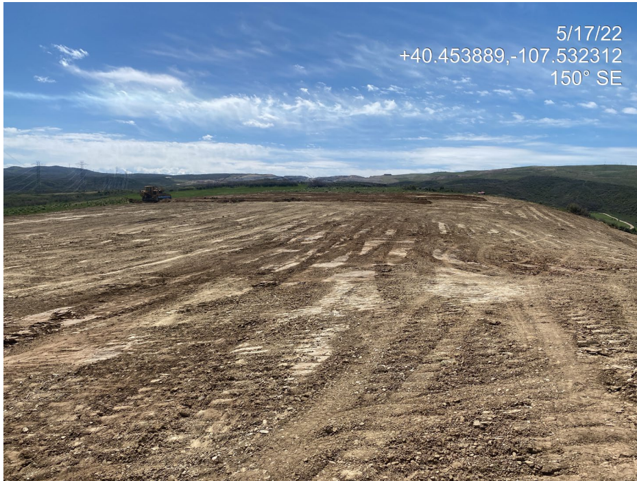
Photo 1. Photo taken from the north of the Location shows an overview of the Location. Final reclamation activities have been initiated. A dozer can be seen in the background replacing topsoil before decompacting the Location.
