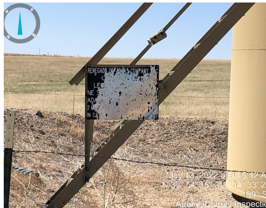
Photo #2 well sign in crude tank is faded and illegible.
