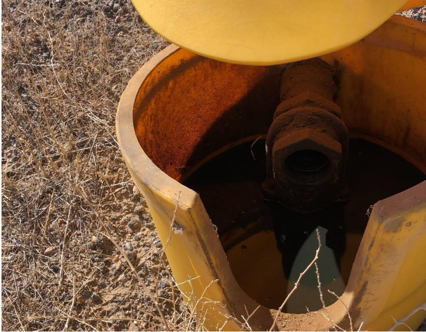
Photo #5 no bull plug in in load-off line
