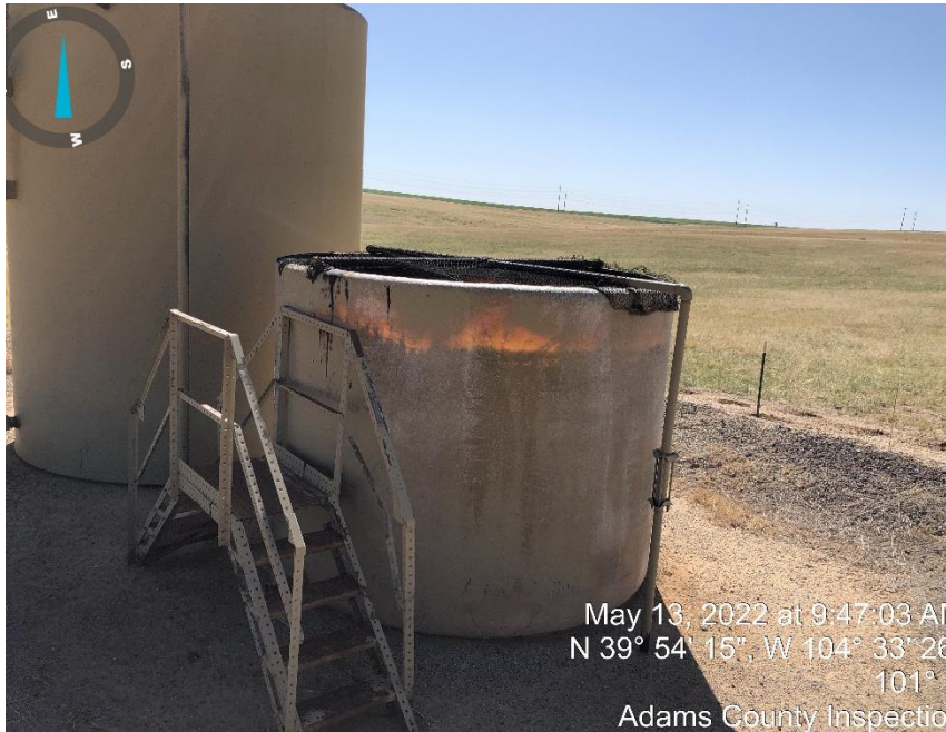
Photo #7 wildlife netting has fallen in to open top tank.
