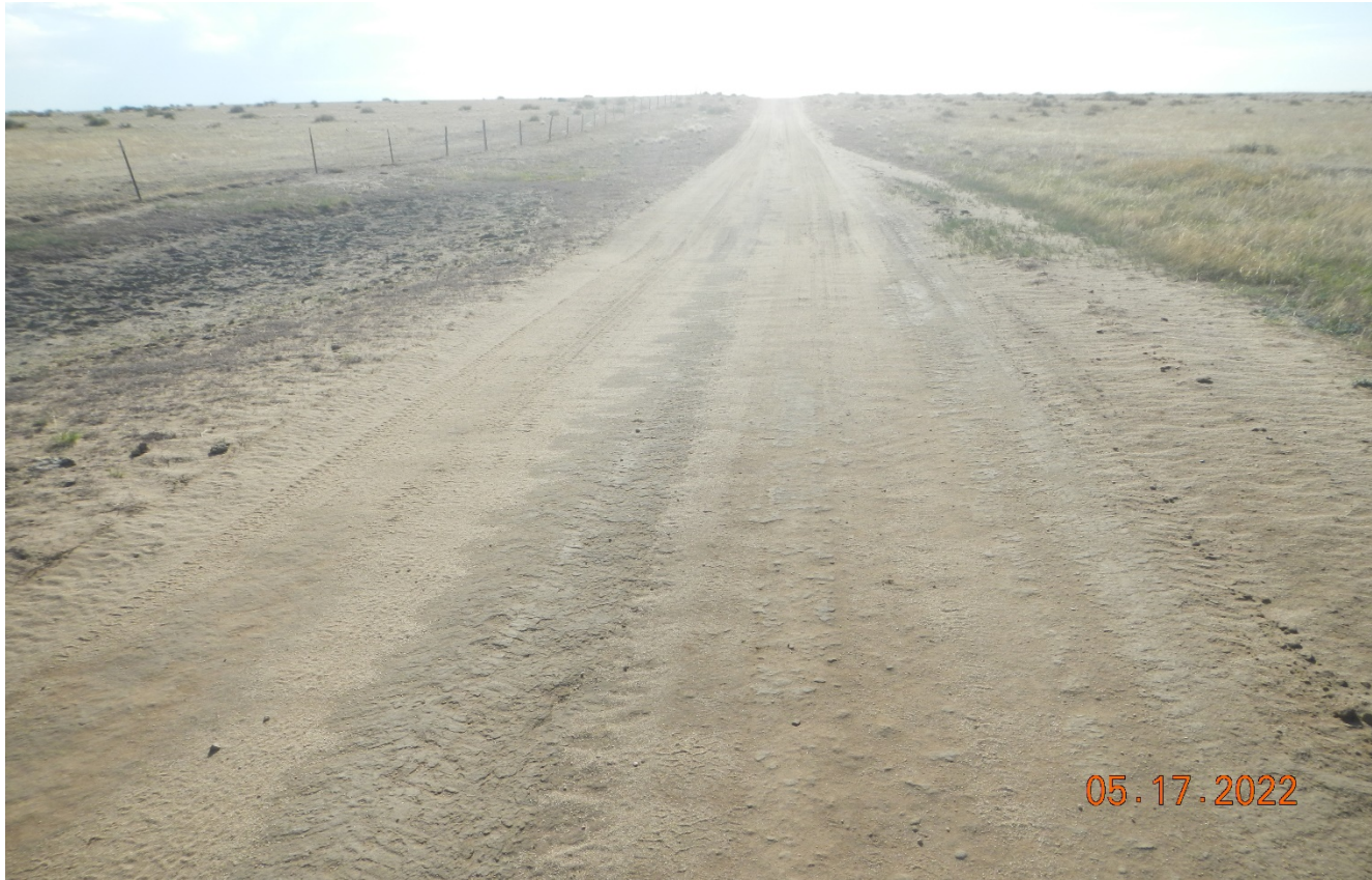
Photo 1. Facing east along the access road. It appears stormwater pool on the road in this area causing vehicles to widen the road. This area needs to be repaired.
