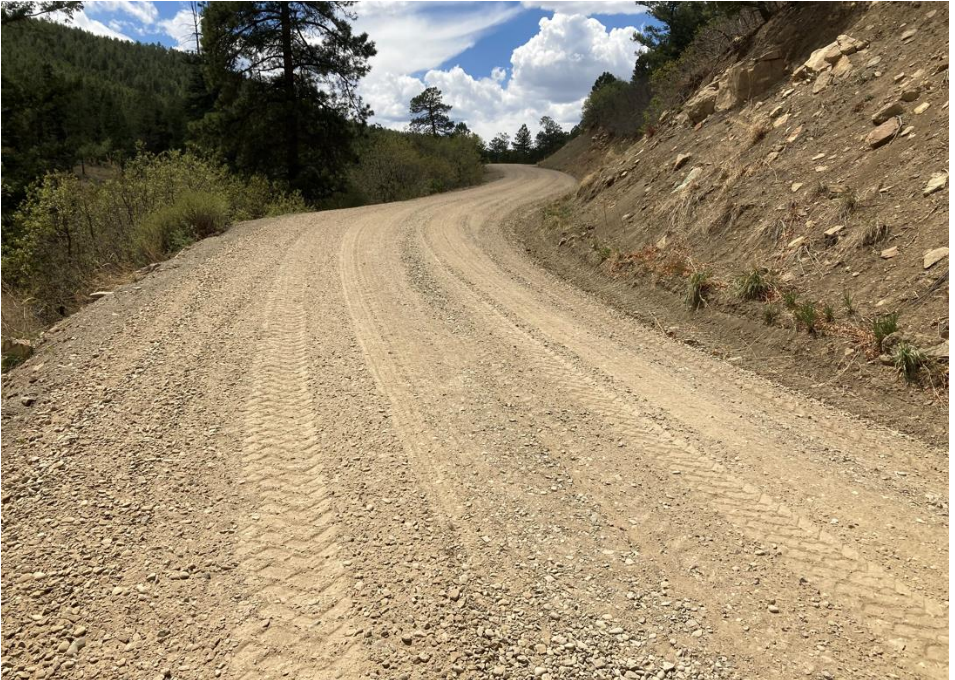
PHOTO 3: THE ROAD SURFACE WAS RE-GRADED TO ELIMINATE THE TIRE RUTS AND STABILIZED.
