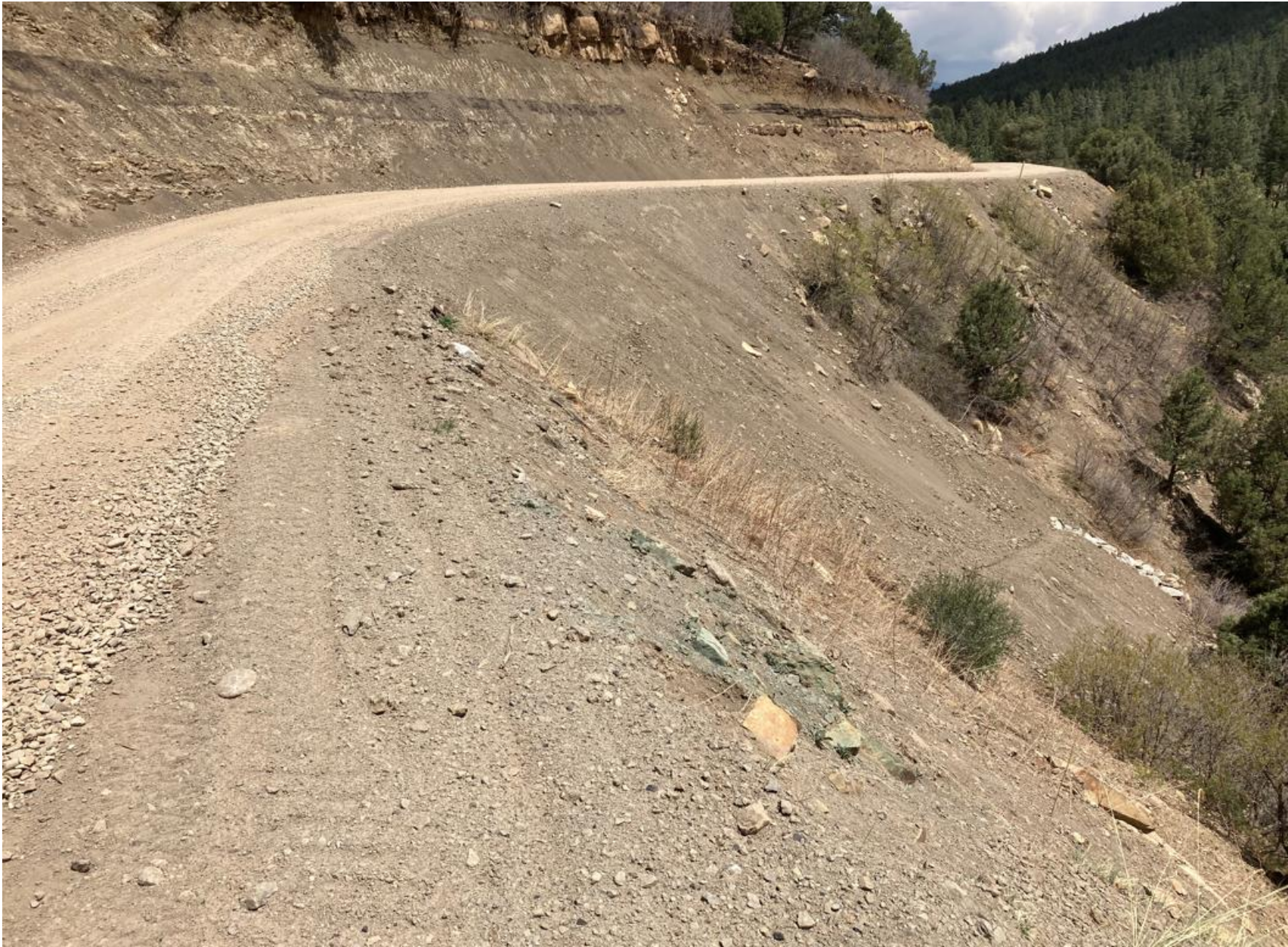
PHOTO 1: THE EROSION OF THE FILL SLOPE ON THE UPPER MAIN LEASE ROAD OF ALAMOSITO WAS REPAIRED. THE DIVERSION DITCH ALONG THE ENTIRE ACCESS HAS BEEN CLEANED OF SEDIMENT AND REDefined TO DIRECT STORMWATER TO CULVERTS. THE FILL SLOPE HAS ALSO BEEN SEEDED USING AN APPROVED CPW SEED MIX TO PROMOTE THE ESTABLISHMENT OF VEGETATION.
