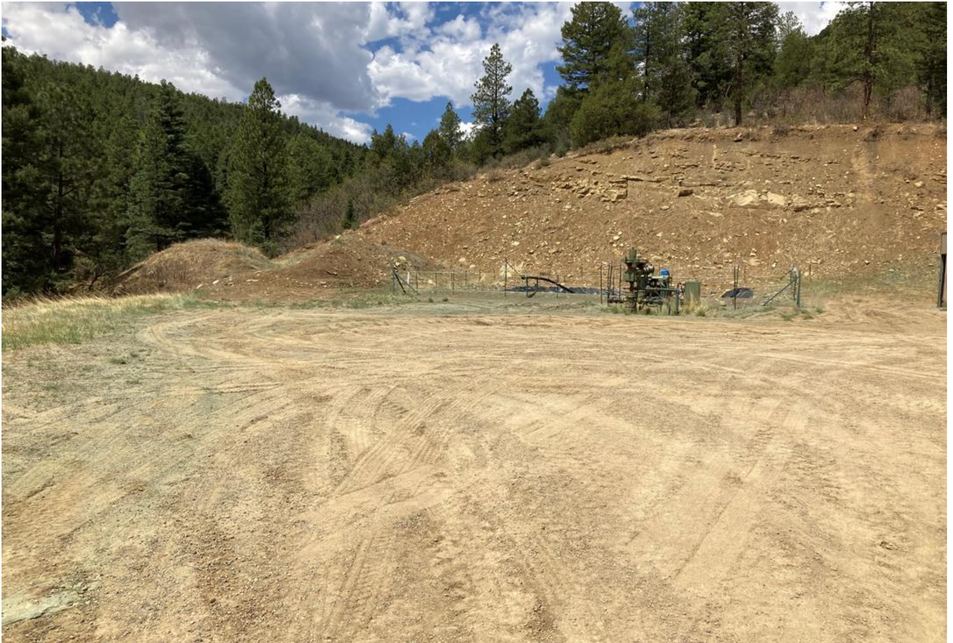
PHOTO 5: THE WELL PAD WAS REGRADED TO KNOCK DOWN THE TIRE RUTS.
