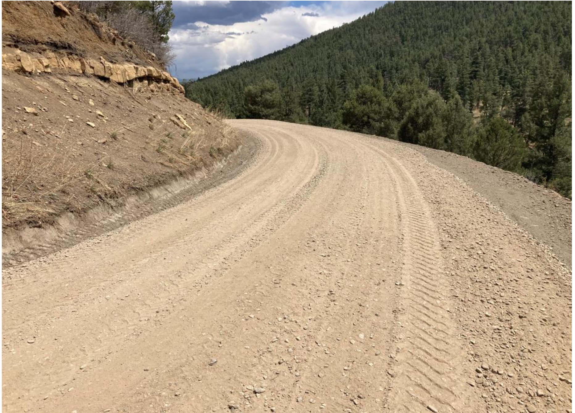
PHOTO 2: THE MAIN LEASE ROAD SURFACE WAS CROWNED TO CREATE SHEET FLOW AND ELIMINATE THE TIRE RUTS. GRAVEL WAS ADDED TO THE ROADWAY SURFACE FOR STABILIZATION.
