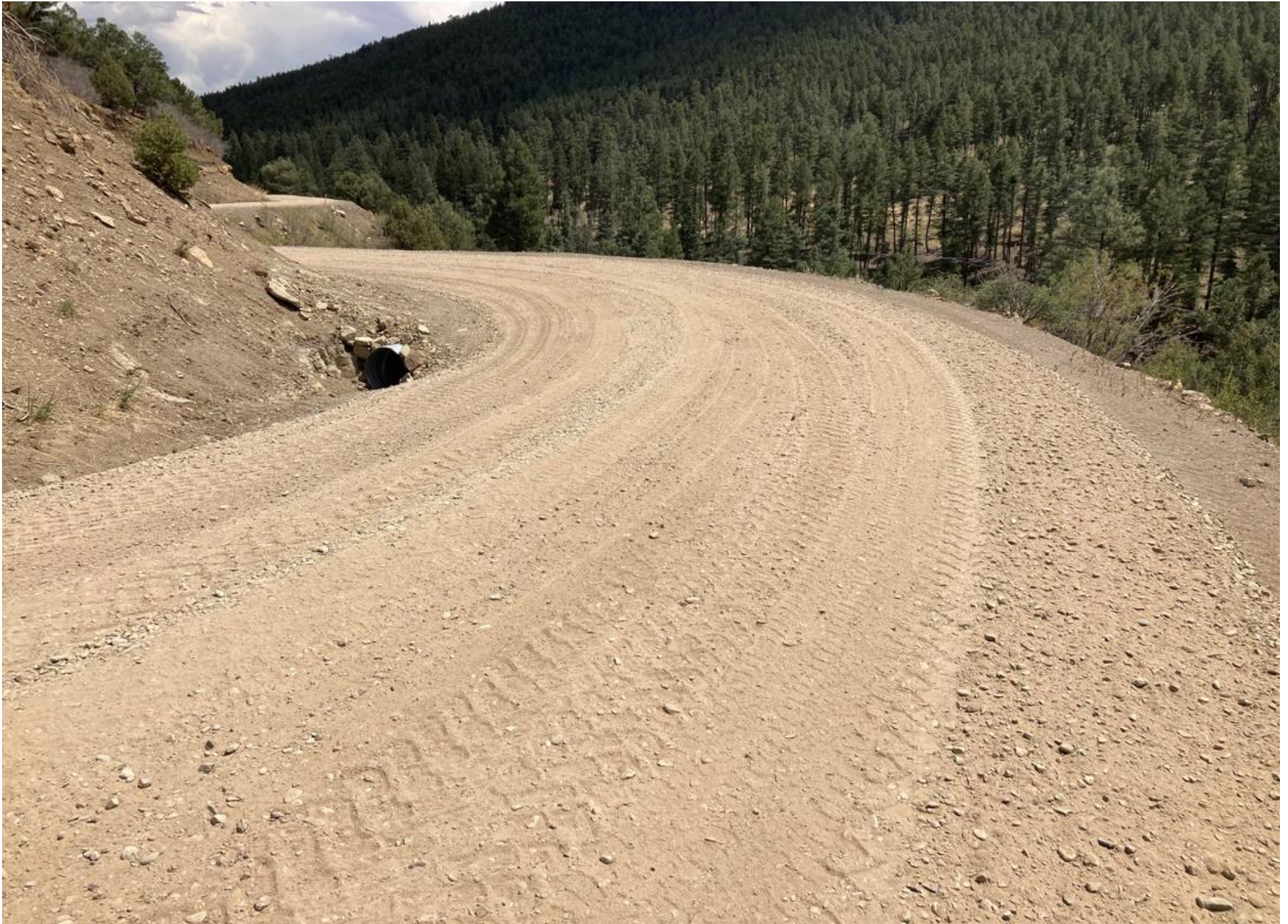
PHOTO 4: THE ROAD SURFACE WAS RE-GRADED TO ELIMINATE THE TIRE RUTS AND STABILIZED.
