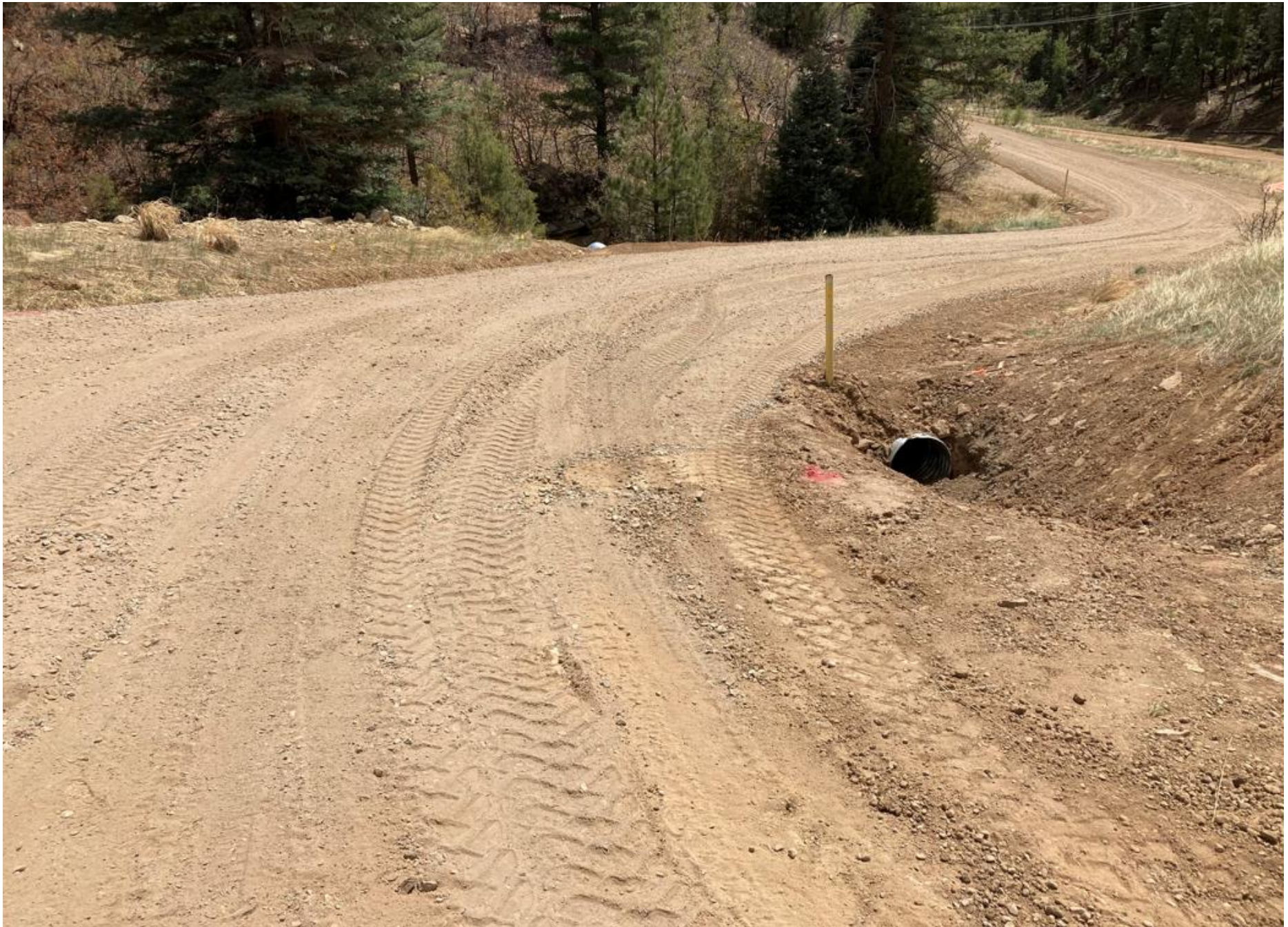
PHOTO 8: A CULVERT HAS BEEN INSTALLED AT THE INTERSECTION BELOW LOCATION. THE DIVERSION DITCH WAS DEFINED TO RECEIVE STORMWATER RUN OFF FROM THE ABOVE ACCESS ROAD AND DIRECT RUN OFF TO THE CULVERT INLET. THE ROAD SURFACE WAS CROWNED TO CREATE SHEET FLOW AND DIRECT SURFACE RUN OFF TO THE CULVERT INLET.
