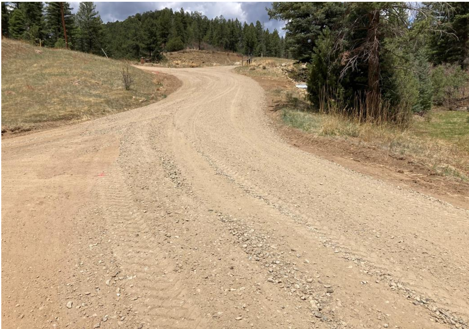
PHOTO 7: THE RUTTING ALONG THE MAIN ACCESS ROAD, AT THE INTERSECTION BELOW THE LOCATION, HAS BEEN REPAIRED AND STABILIZED.
