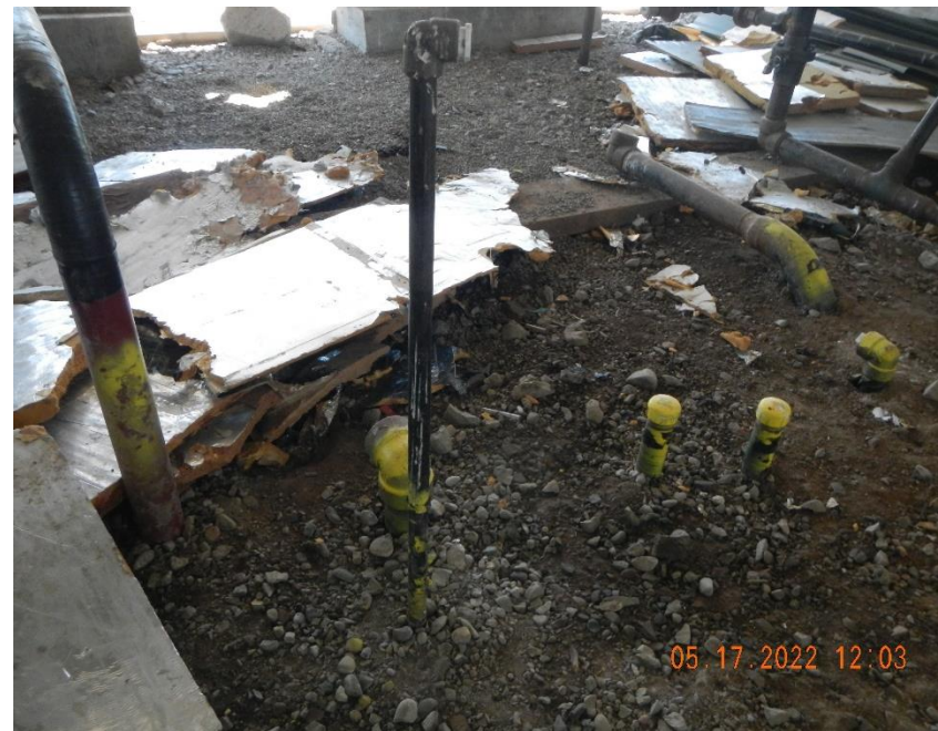
Staining of ground surface under shed that surface equipment was removed from. Unused equipment on location. Unused 15 flowline risers.
