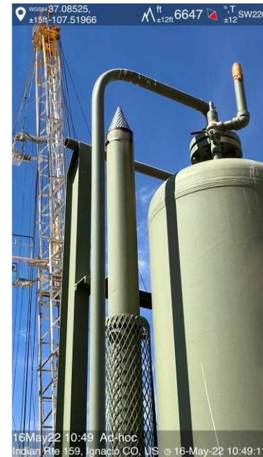
IMG 10 Separator vent stack with screen
