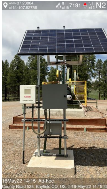
IMG 11 Pump control panel
