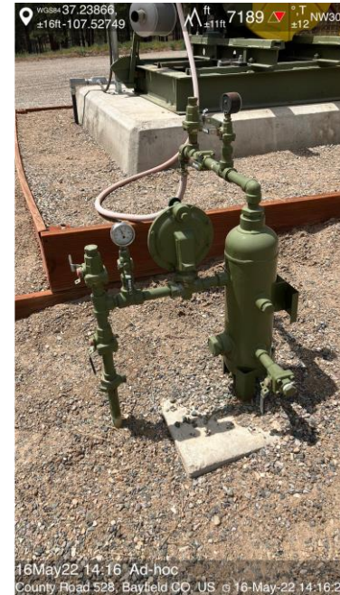
IMG 12 1" flow line to pump jack generator
