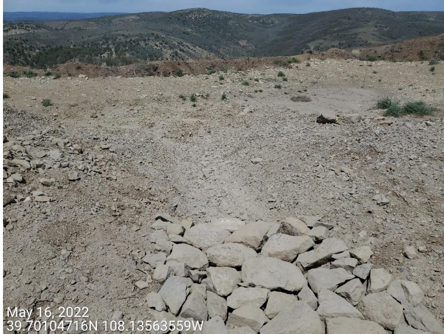
Photo 9: Photos taken from the sediment trap on the north end of the Location. Inlet at the sediment trap/pond on the north end of the Location does not appear to be properly engineered; gully erosion/degradation becoming apparent at the inlet/control.
