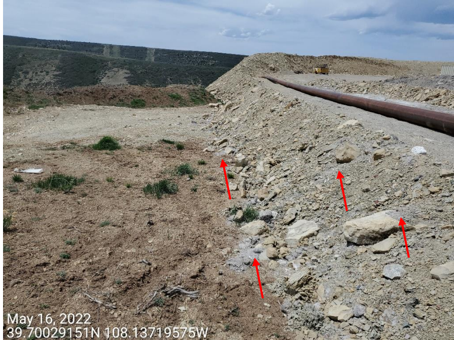
Photo 12: Continue from photo 10/11. Photo shows impacted materials observed outside of containment. Operator does not appear to have properly cleaned spill. Photo left also shows proximity of spill to the sediment trap/basin on the south end of the location, as well as the topsoil used as the berm for the trap.
