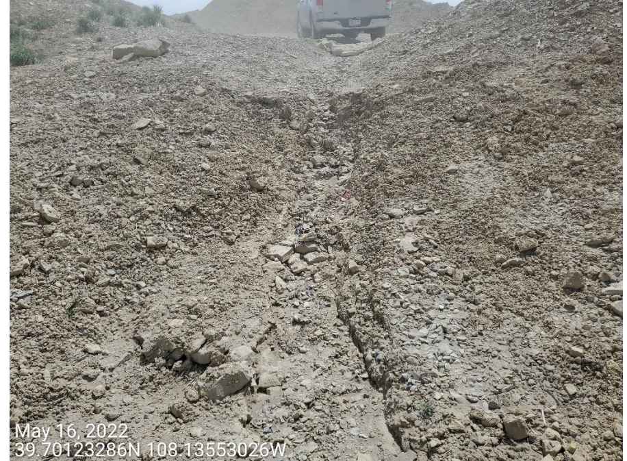
Photo 9: Photos taken from the sediment trap on the north end of the Location. Inlet at the sediment trap/pond on the north end of the Location does not appear to be properly engineered; gully erosion/degradation becoming apparent at the inlet/control.
