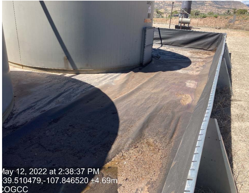
Staining and missing cap/plug
