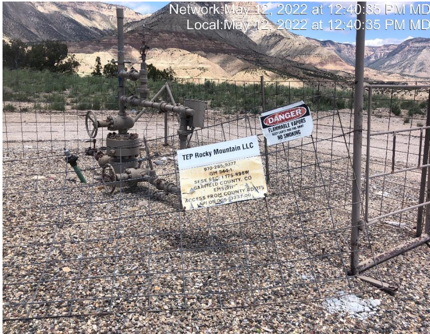
Photo #6689 Wellhead sign weathered and not legible.
