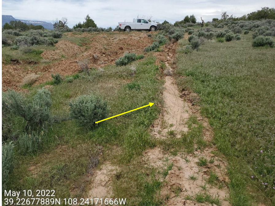
Photo 8: Photos examples of erosion degradation and sediment transport and deposition observed at access road. Stormwater and erosion control measures to minimize erosion, degradation and sediment transport and deposition (Lighter soils) at and from the access road remains missing or insufficient.
