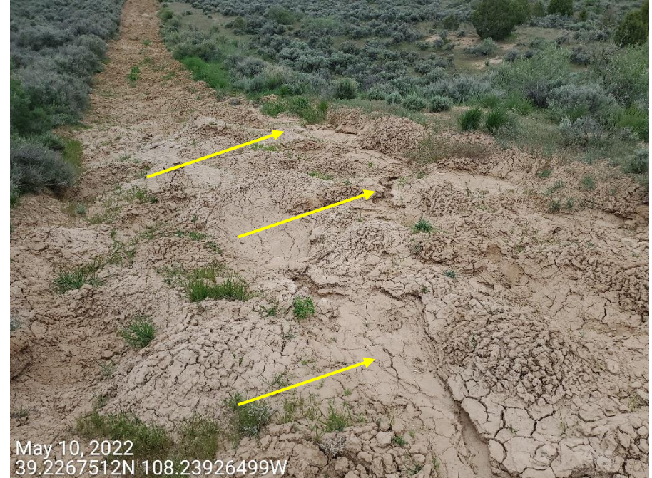
Photo 8: Photos examples of erosion degradation and sediment transport and deposition observed at access road. Stormwater and erosion control measures to minimize erosion, degradation and sediment transport and deposition (Lighter soils) at and from the access road remains missing or insufficient.
