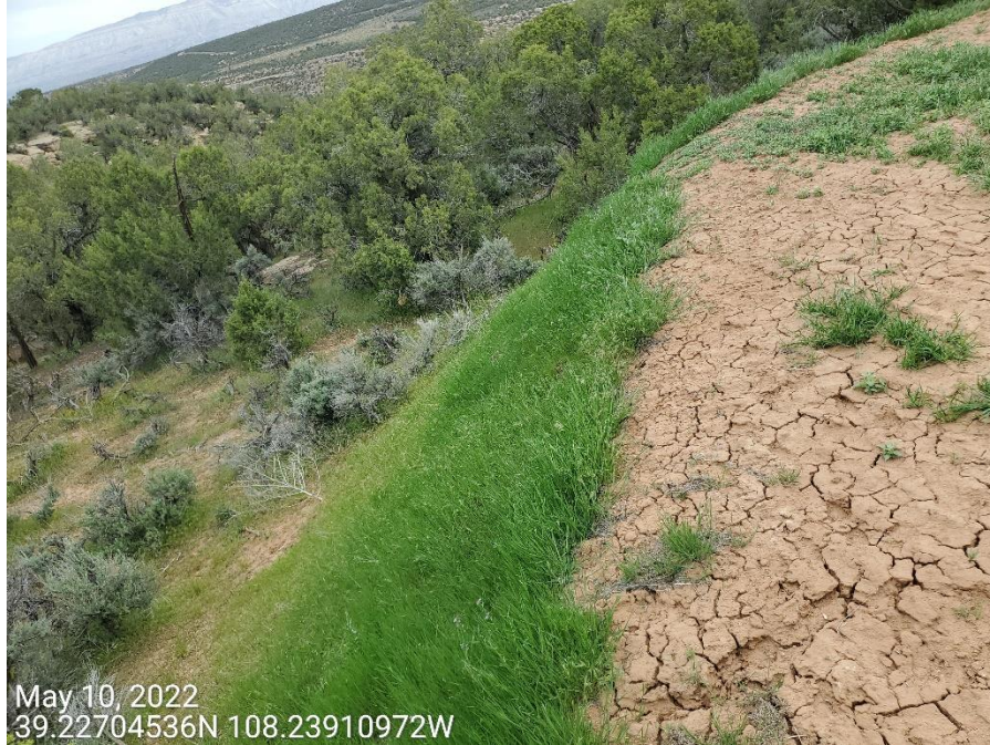
Photo 3: Photo shows fill slopes remaining; location has not been recontoured and regraded.
