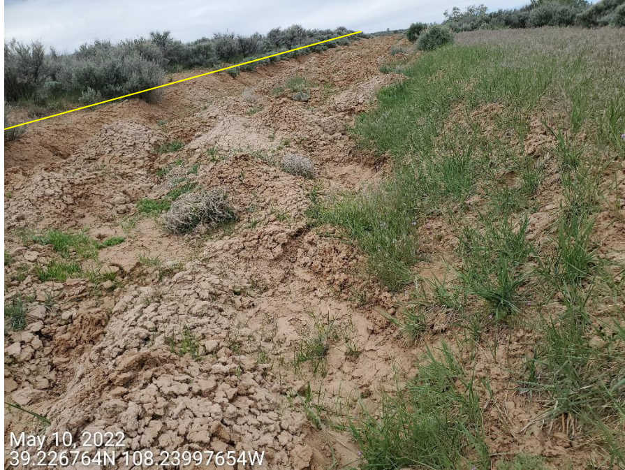
Photo 7: Photos taken from the access road. Photos show access road has not been properly recontoured/regraded to the original relative grade, and to that of the reference. Yellow line represent top grade of the adjacent areas.
