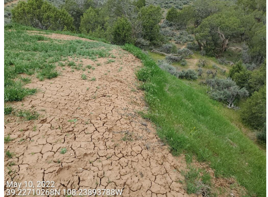
Photo 3: Photo shows fill slopes remaining; location has not been recontoured and regraded.
