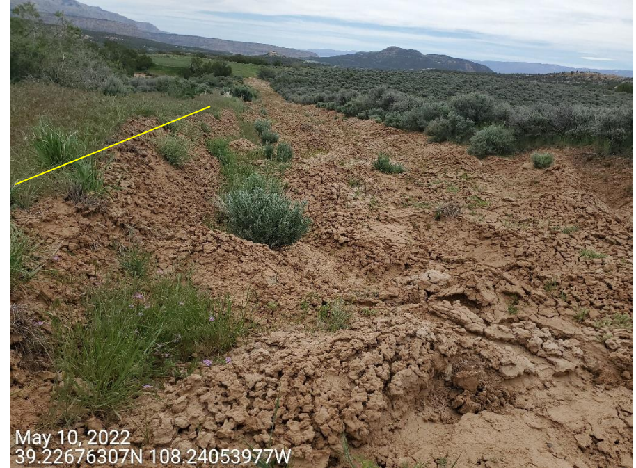
Photo 7: Photos taken from the access road. Photos show access road has not been properly recontoured/regraded to the original relative grade, and to that of the reference. Yellow line represent top grade of the adjacent areas.
