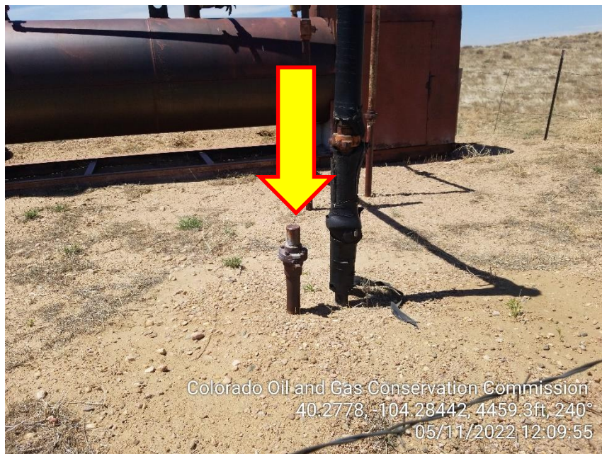
Photo 5 – Unmarked Riser
