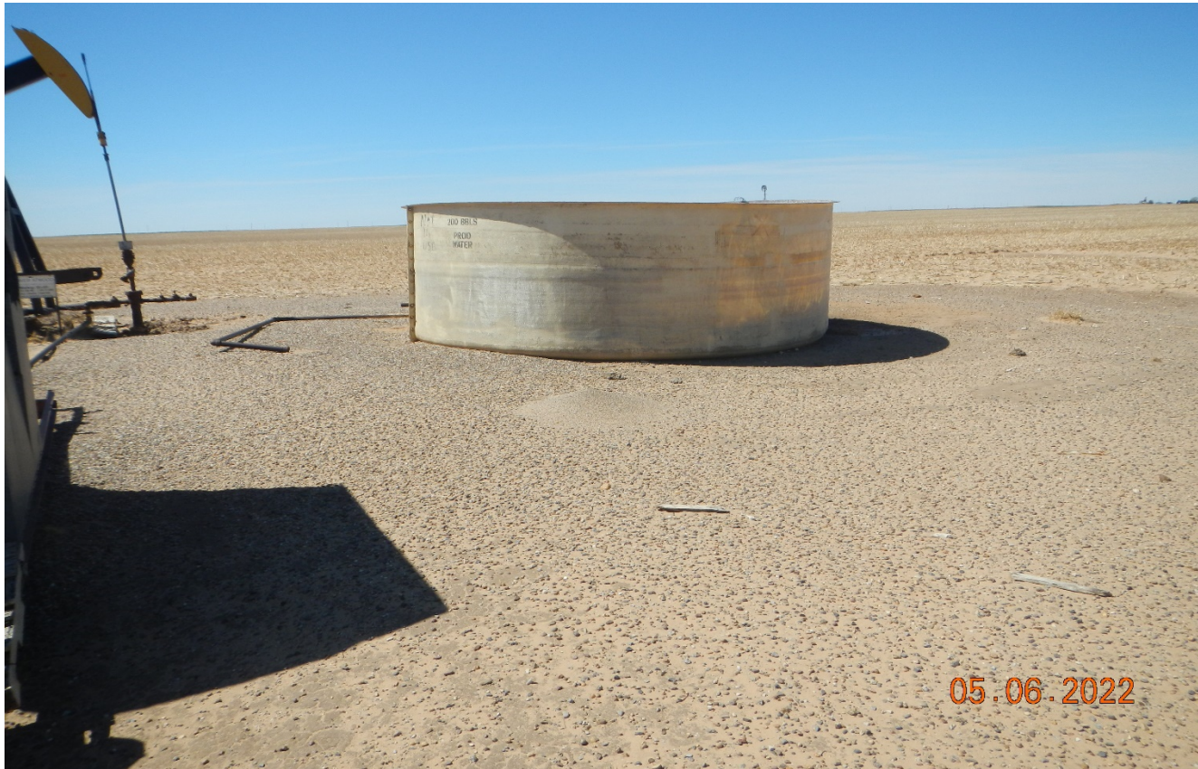
Photo 2. Missing tank NFPA labeling and missing INFO per 605.h.. Secondary containment is inadequate to contain 150% of the volume of the tank. Previous corrective action not completed.
