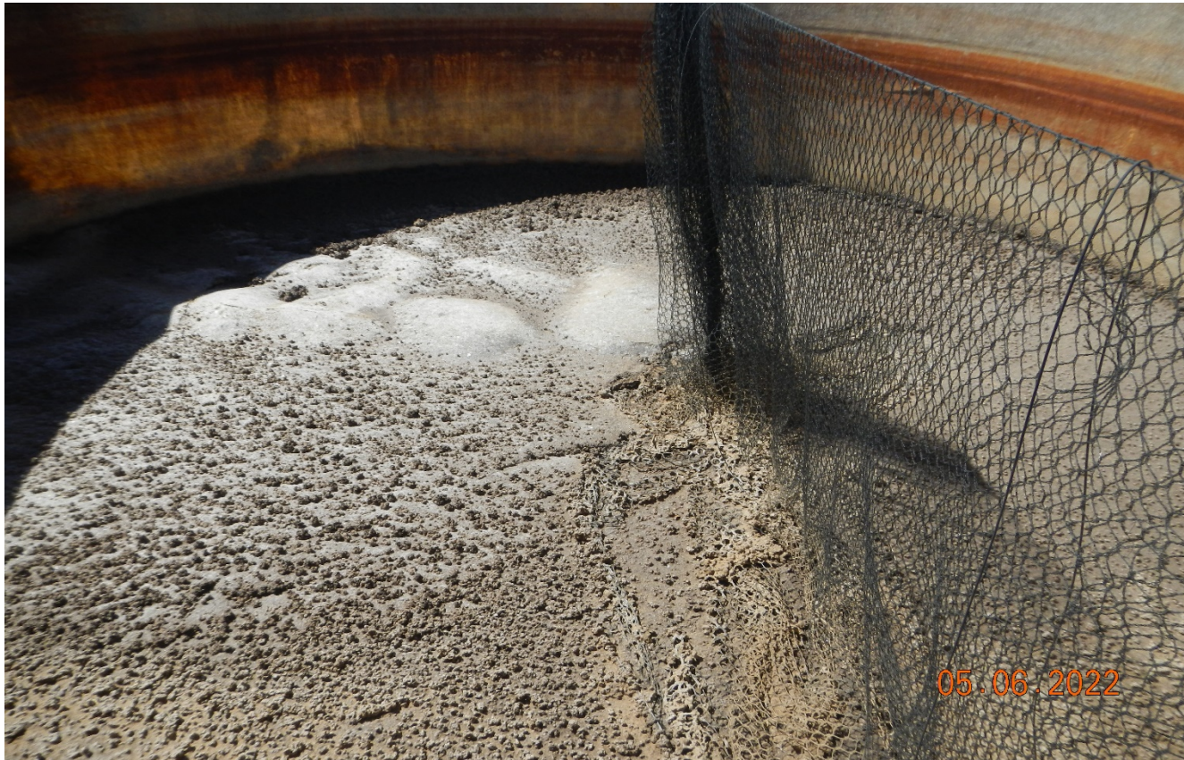
Photo 3. View of fluids inside the tank. Tank is labeled Produced Water. It appears to be solidified salty produced water. The netting on the tank is in disrepair. Previous corrective action not completed.
