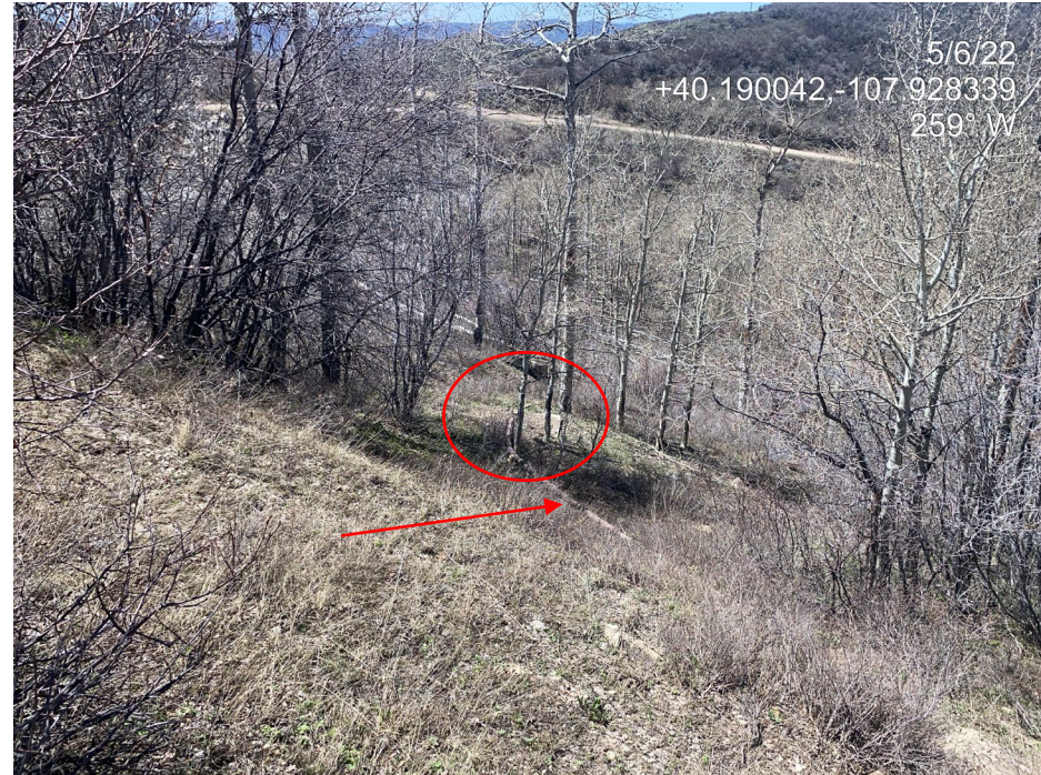
Photo 6. Photo taken from the northwest of the Location shows a flowline (arrow) and pad (circle) which will need to be removed during final reclamation.
