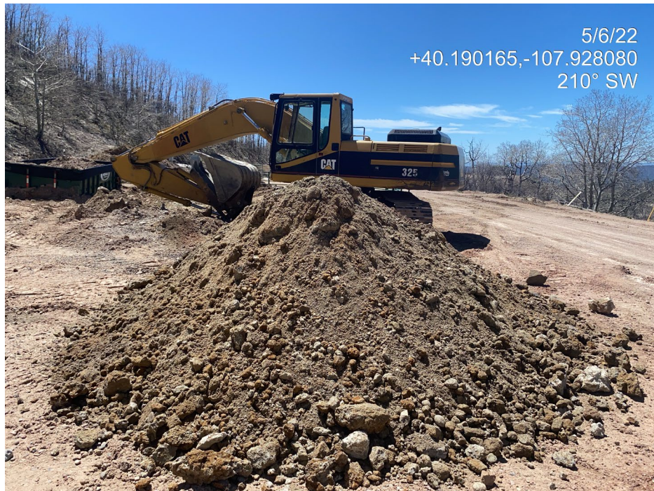
Photo 3. Photo taken from the northeast of the Location shows a pile of material excavated from around the well. BMPs to prevent the E&P waste from migrating off the Location were not present.
