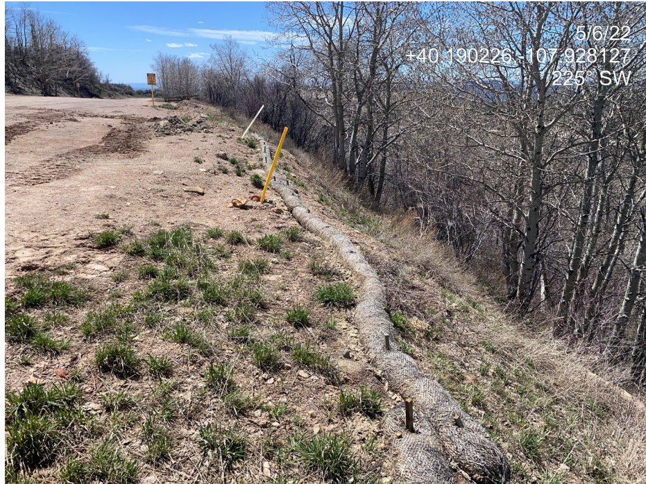
Photo 7. Photo taken from the northwest of the Location shows a straw wattle, which is presently in proper functioning condition to manage stormwater on the Location.
