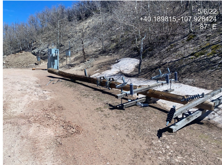
Photo 8. Photos shows power lines being decommissioned at the Location.
