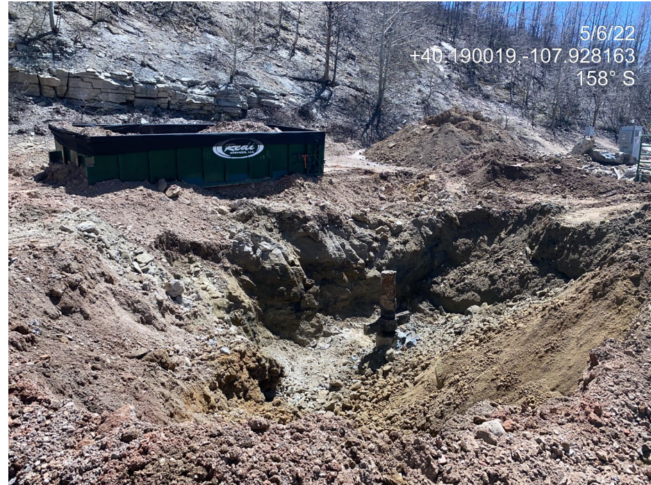
Photo 2. Photo taken from the northeast of the Location shows the excavated well. A strong hydrocarbon odor was present. Photos also shows the sides of the pit may be too steep to allow wildlife escape and fencing to prevent access does not completely enclose the excavated area.
