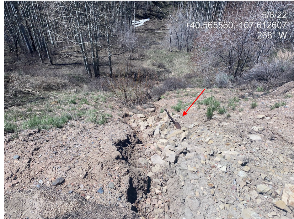
Photo 7. Photo taken from the west of the Location shows gully erosion. Photo also shows buried pipe which will need to be removed during reclamation.
