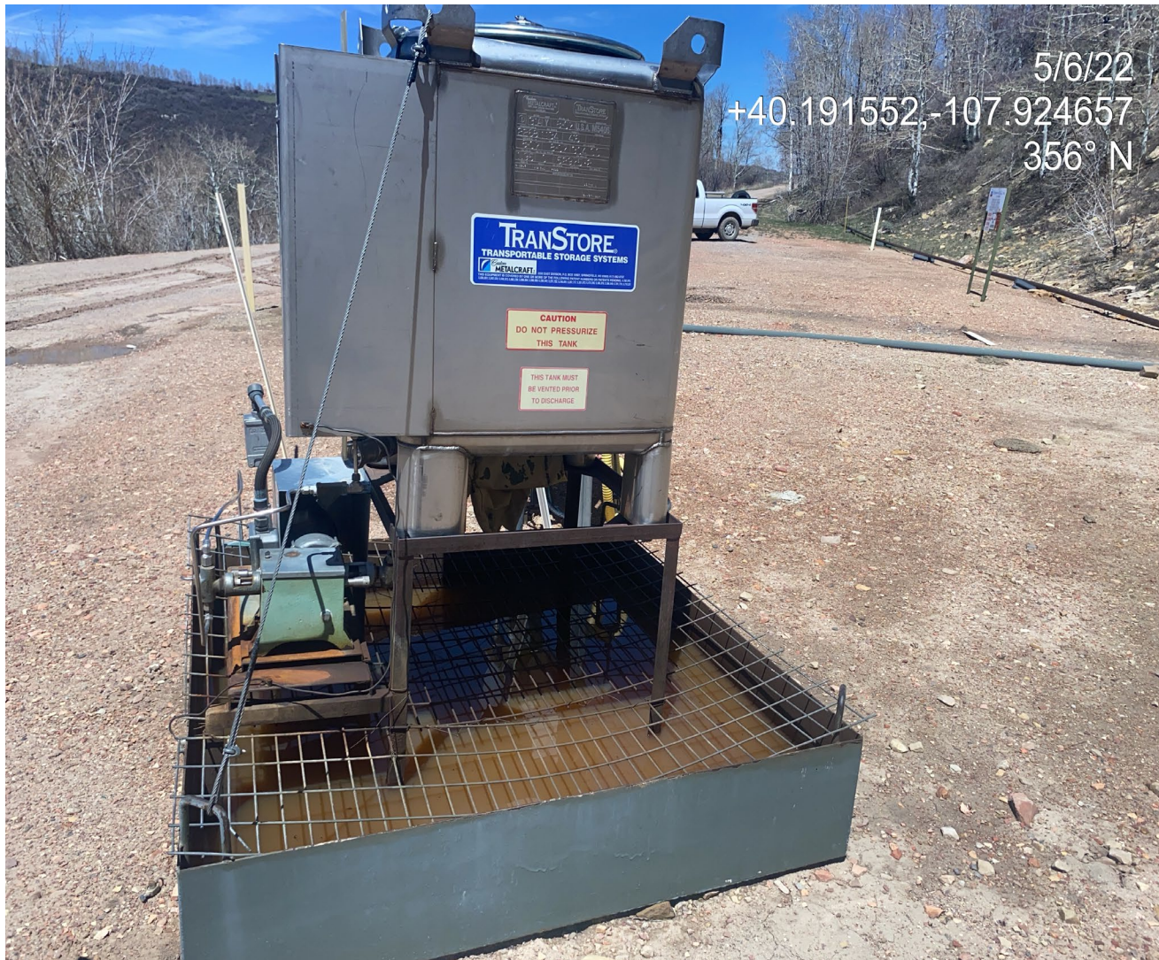
Photo 3. Photo shows a secondary containment BMP filled with fluid. Wildlife protection BMPs to enable wildlife egress are missing or insufficient.
