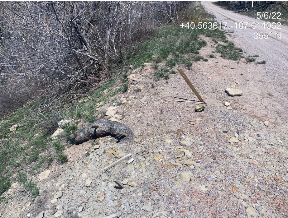
Photo 4. Photo taken from the west of the Location shows a straw wattle not in proper functioning condition. Erosion is occurring throughout the slope at the western perimeter of the Location. Sediment leaving the Location appears to be causing degradation to areas offsite.
