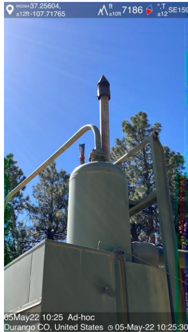
IMG 05 Separator vent properly screened
