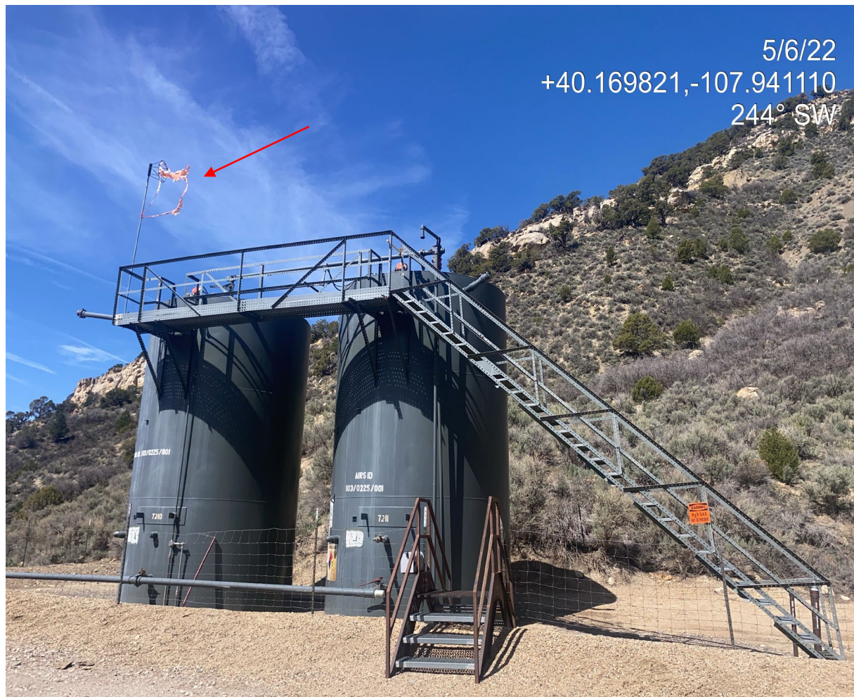
Photo 3. Photo shows the wind direction indicator in disrepair.
