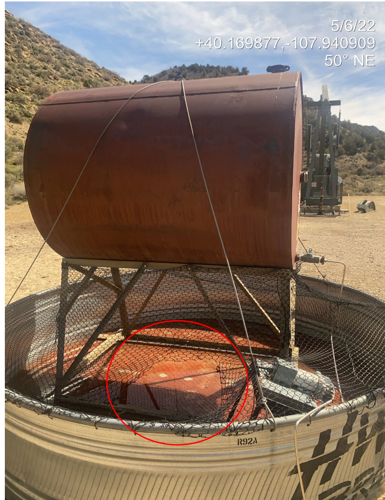
Photo 6. Photo taken from the north of the Location shows BMPs to prevent wildlife entry to the methanol tank secondary containment are in disrepair.
