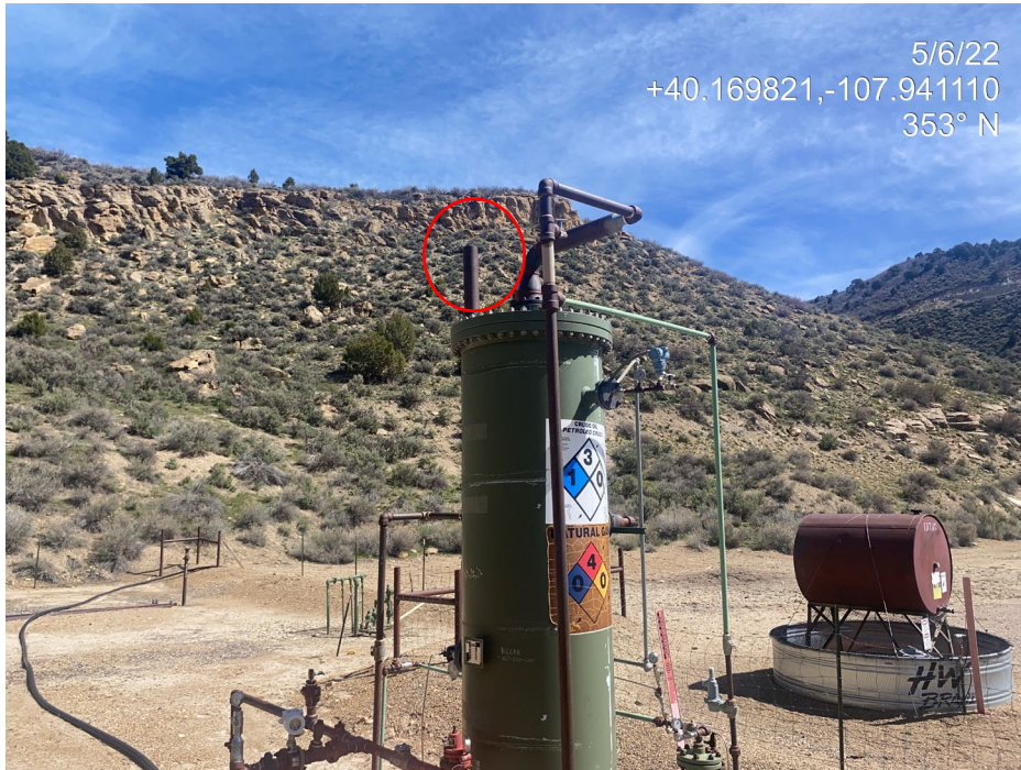
Photo 4. Photo shows bird protection devices are missing or insufficient on pipe equipment to the northwest of the Location.
