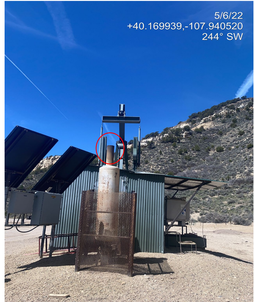
Photo 5. Photo shows bird protection devices are missing or insufficient on pipe equipment to the northeast of the Location.
