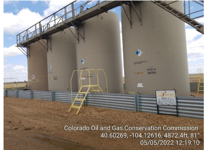
Photo 10 – Tank Battery – Capacity Labels Missing
