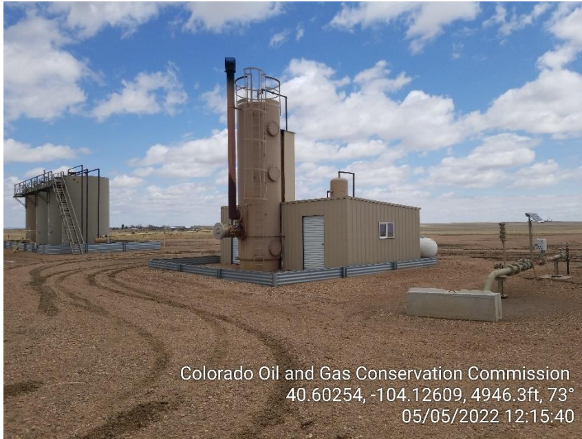
Photo 1 – Heater Treater and Gas Meter
