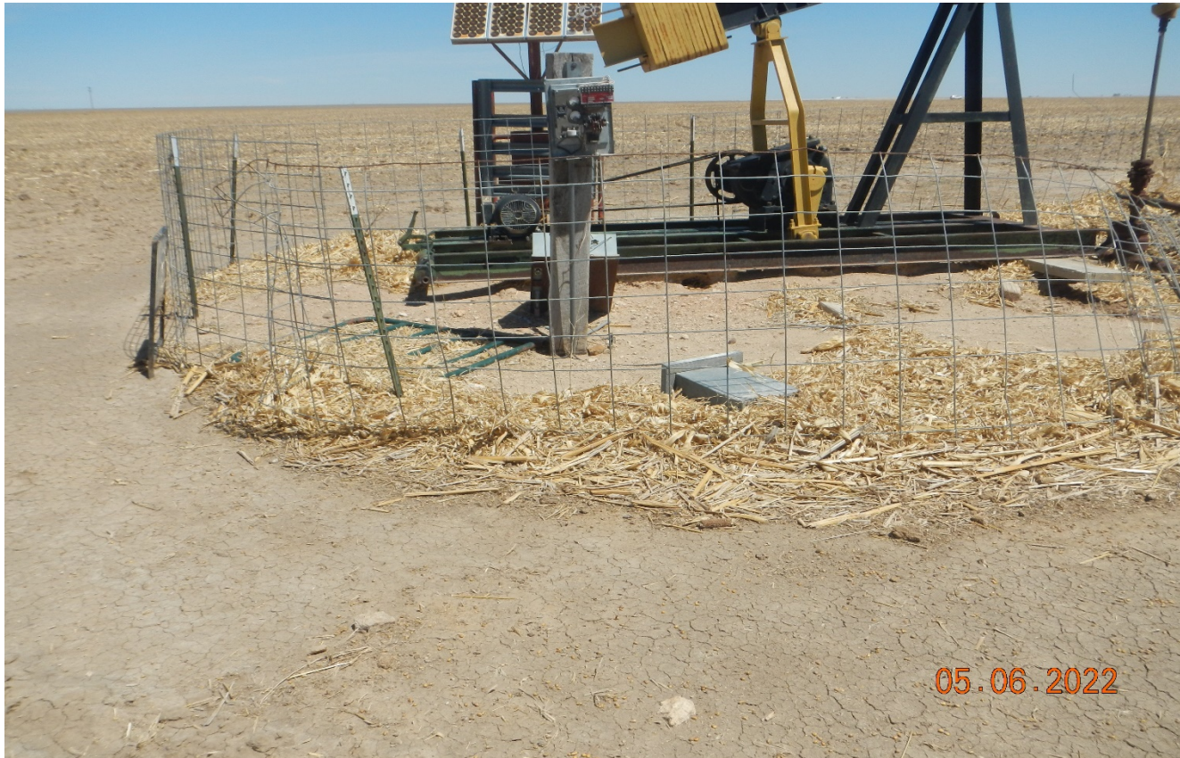
Photo 5. There is a gate and unused supplies lying on the ground. There is no cover for the electric utility which is a safety concern.
