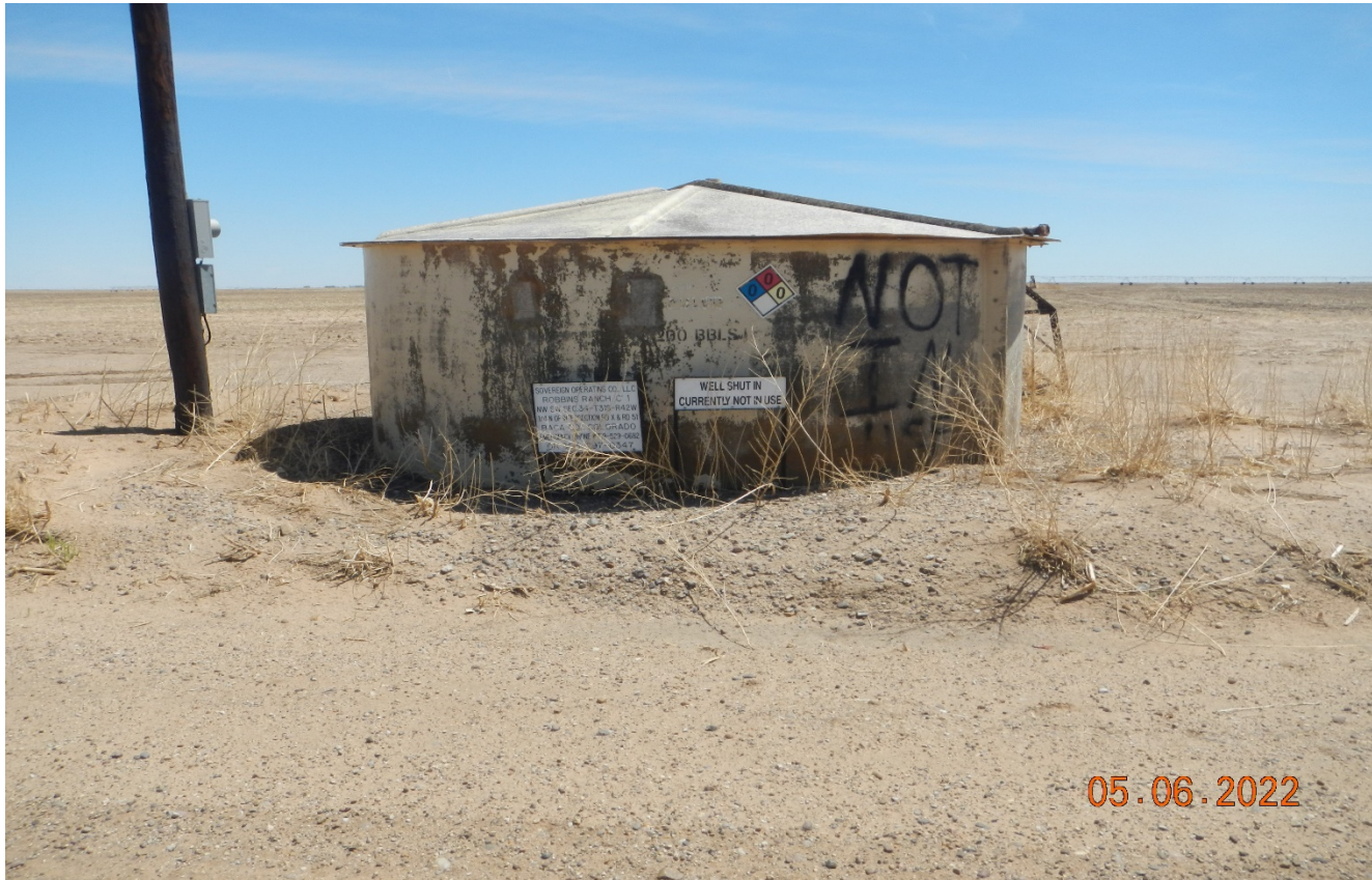
Photo 1. Facing east toward the tank battery along the access road. Sign does not reflect current Operator or emergency contact INFO. If take is not in use it must be removed. Tank berm is inadequate.
