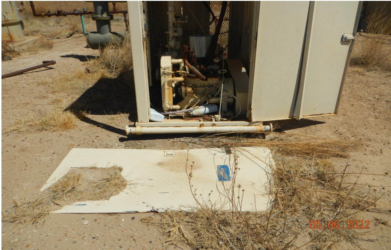
Photo 6. There is equipment not maintained on location. Door has fallen off this shed. Previous corrective action is not completed.
