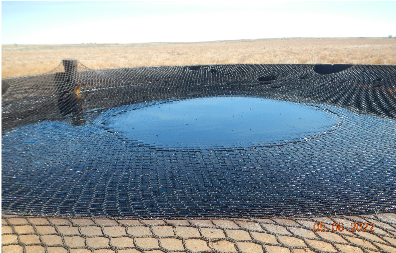
Photo 9. The liquid in the tank is near the top which could spill over. The netting is not adequate to prevent wildlife entry. Previous corrective action is not completed.
