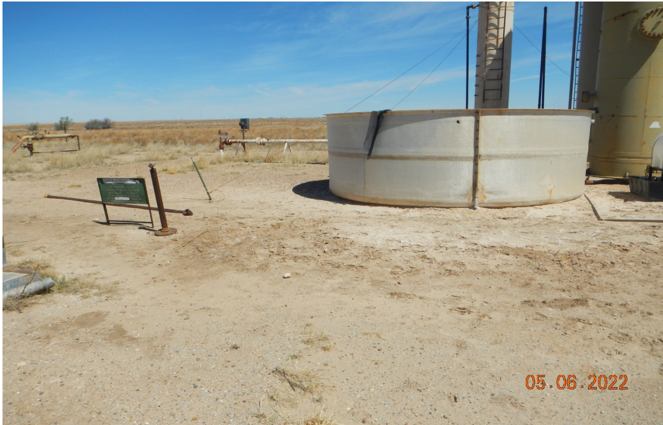
Photo 4. Facing toward the open top tank. It appears the tank has previously leaked due to white stained soil. There is no secondary containment around the tank. There is no signage on the tank. Previous corrective action is not completed.
