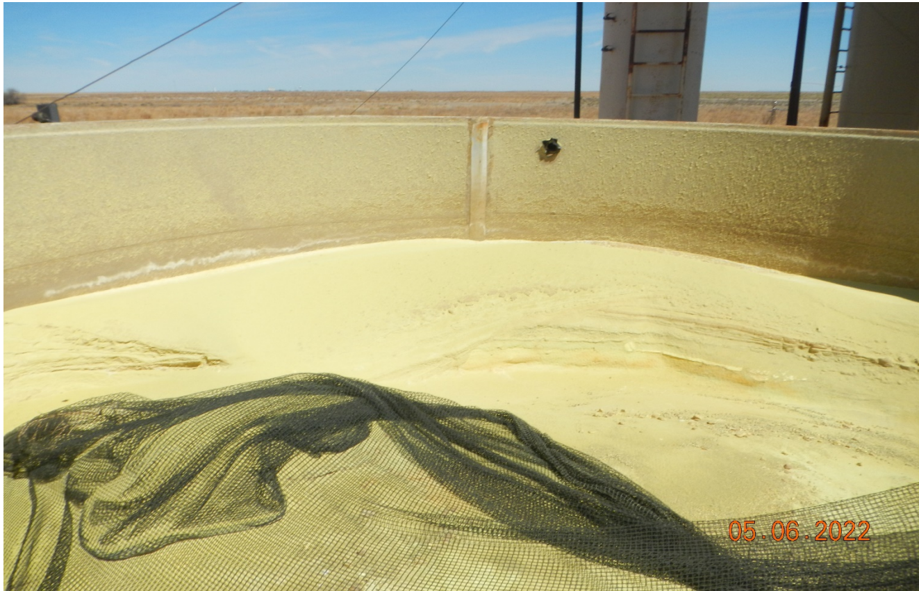
Photo 5. The netting over the tank is not installed. Previous corrective action is not completed.
