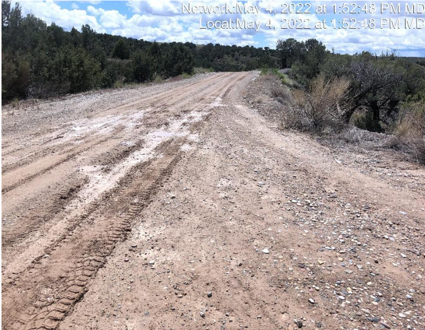
Photo #6616 Insufficient tracking control at entrance to location.
