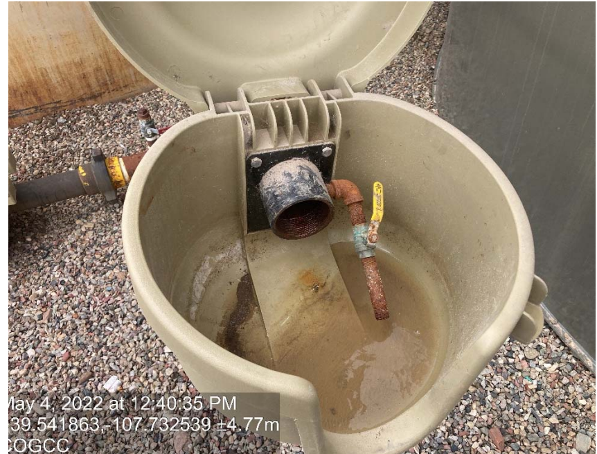
Valve on tank missing cap/plug
