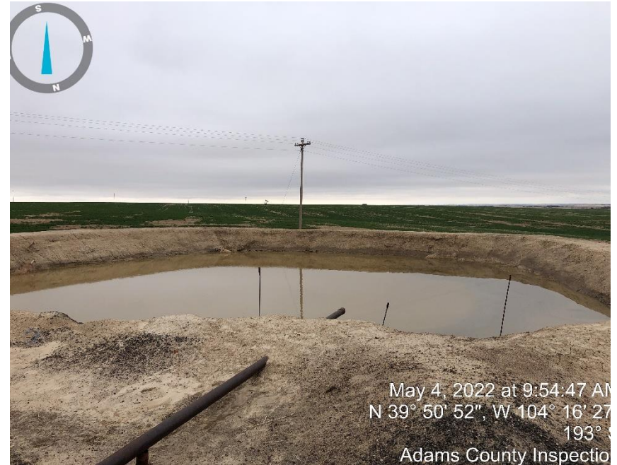
Photo #8 Produced water pit.
