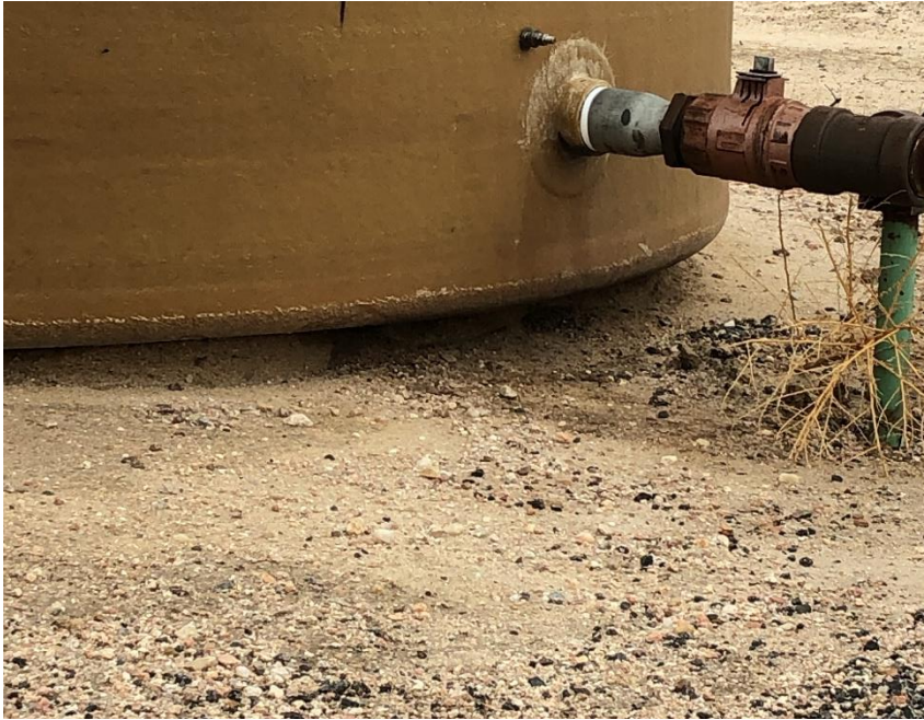
Photo #7 gap under produced water tank.
