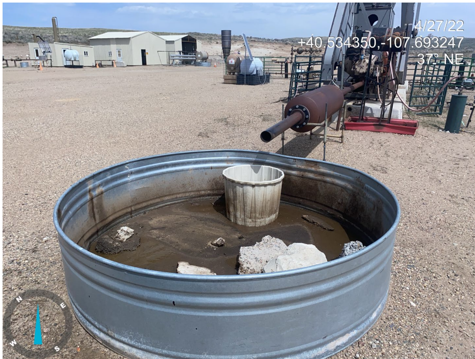
Photo 22. Photos show wildlife protection equipment to prevent wildlife access to secondary containment is missing or insufficient. No safety labeling applied identifying fluids within containers in both photos.
