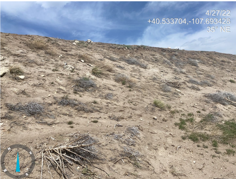
Photo 12. Photos taken from the fill slope at the south of the Location shows wind erosion occurring on unprotected soils. Vegetation on the slope is sparse and dominated by annual undesirable plant species/weeds.
