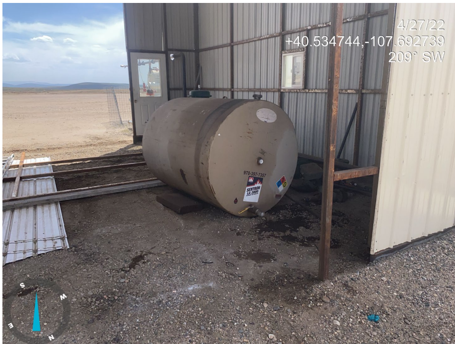
Photo 28. Photos show stained soils and unused equipment throughout the compressor shed Located at the north of the Location.
