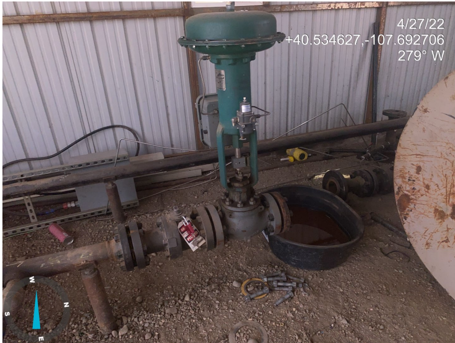
Photo 27. Photos shows unused equipment, tools etc. throughout the compressor shed Located at the north of the Location. Photo also shows wildlife protection equipment to prevent wildlife access to the fluid filled container is missing or insufficient. No safety labeling identifying the fluid.
